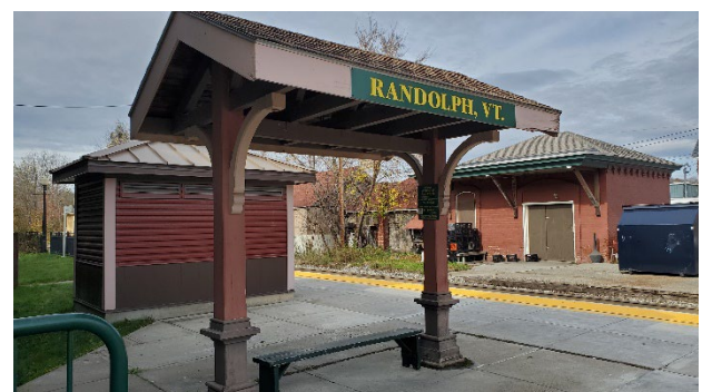
Figure 19. Waiting area at Randolph Train Station
