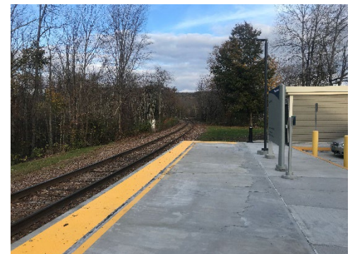
Figure 12. Current Amtrak Platform
