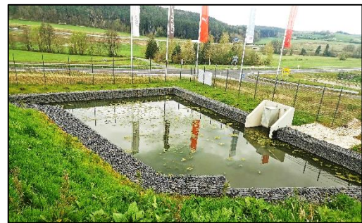
Rainwater retention basin at the distribution center in Geiselwind.
