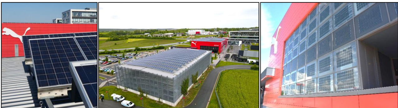
Solar panels on top of the headquarters' parking garage and stores and in the facade of the store in Herzogenaurach.
