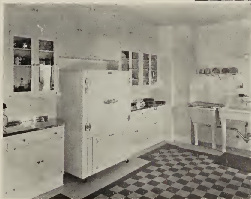
Typical kitchen and pantry layout at 993 Fifth Avenue, New York City Emery Roth, Architect
