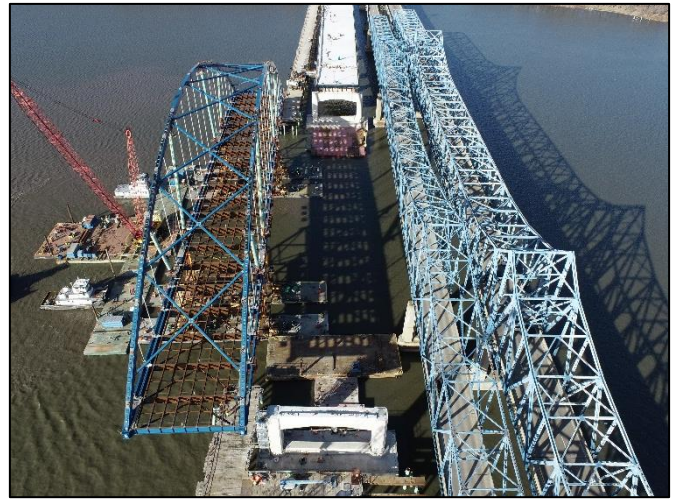
McClugage Bridge arch placement
