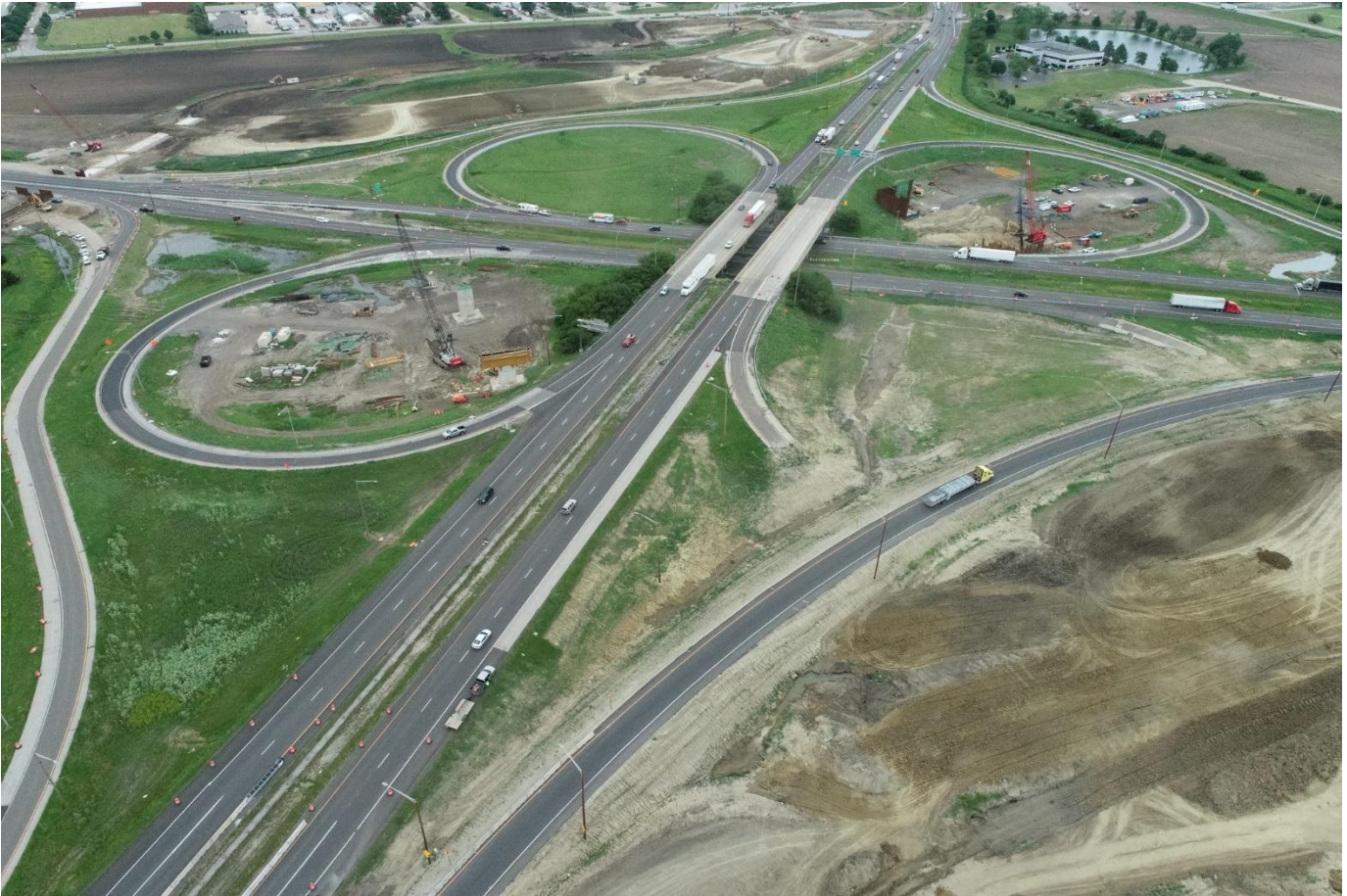
I57-74 interchange construction
