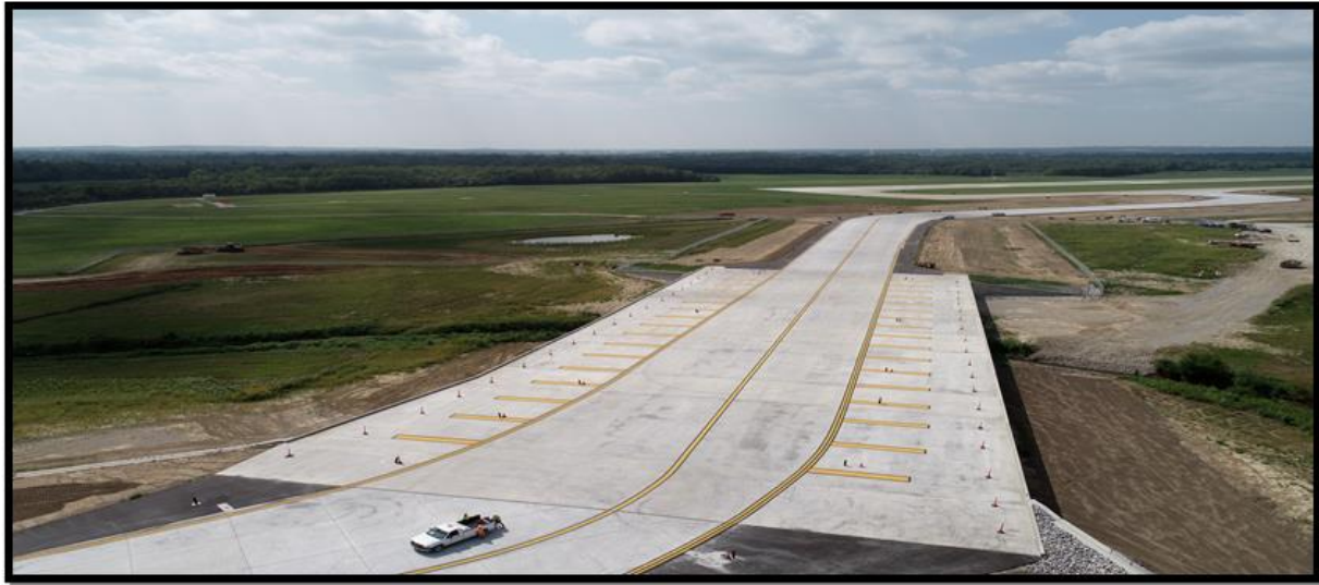
MidAmerica St. Louis Airport Taxiway Lima
