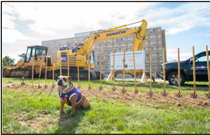
Construction Site at Western Illinois University Performing Arts Center
