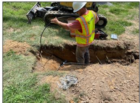
Fiber Broadband Installation
