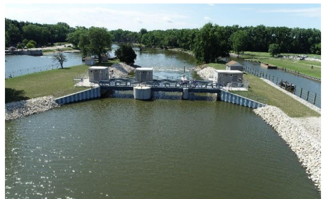
Stratton-Bolger Gate Control Improvements
