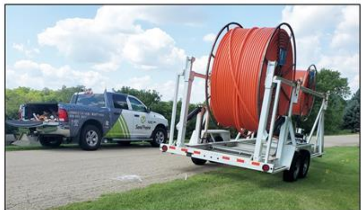
Installation truck and fiber conduit
