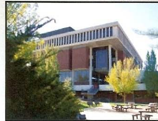
Science Laboratory Building
