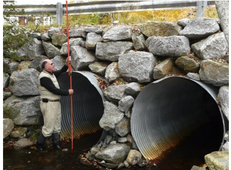
▲ Heavy precipitation to some locations leads to peaks of increased stormwater runoff. Local water managers are assessing their infrastructure's capacity to accommodate sudden heavy flows and prevent flash flooding.
