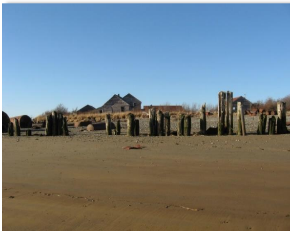
Ward Cove Packing, Bristol Bay Alaska -view of the Graveyard Point cannery from the beach. Note historic buildings, retorts, and numerous 55 gallon drums. (Photo Erin Gleason/ ADEC)
