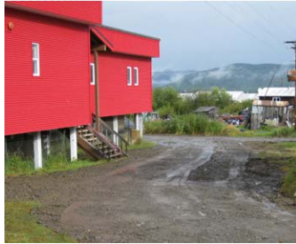
Section of the road by Kaltag School (left) that was excavated and backfilled. Plot of contaminated soils (right) from the Kaltag School being treated by phytoremediation (Photo/DEC)
