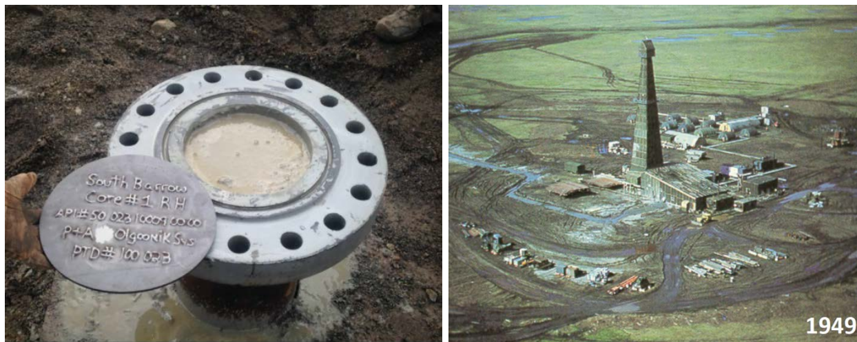
Plugging of South Barrow Core #1, prior to welding cap, during 2016 field season (left) (Photo/Olgoonik Construction Services), Fish Creek No. 1 well operations during summer 1949 (right) (Photo/George Gryc)
