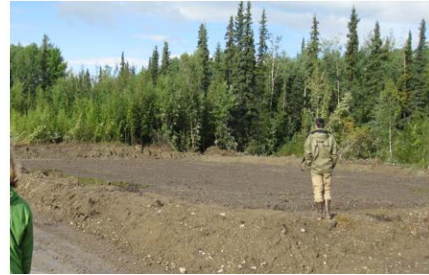
Section of the road by Kaltag School (left) that was excavated and backfilled. Plot of contaminated soils (right) from the Kaltag School being treated by phytoremediation (Photo/DEC)
