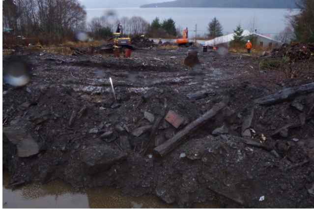
Removal action includes battery parts mixed with the soil and drums of petroleum waste, 2016. (Photos/DEC- Bruce Wanstall)
