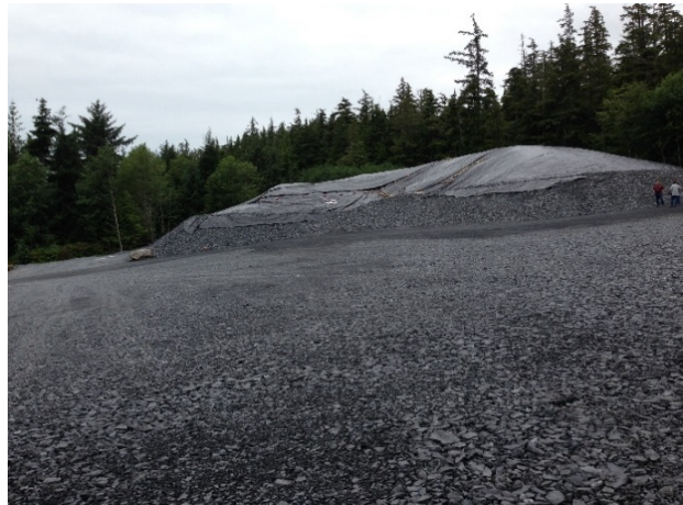
Soil stockpile at the Wrangell Junkyard site. The pile will be moved to an approved monofill, 2016 (Photo/DEC- Bruce Wanstall)
