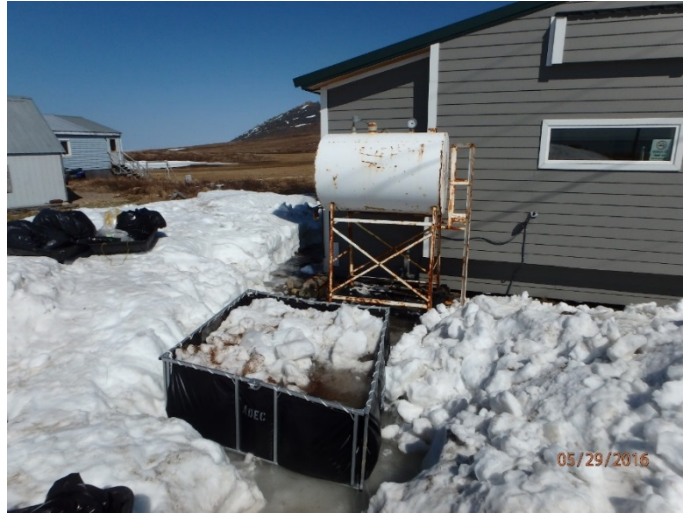
The DEC fold-a-tank was used to contain oil and contaminated snow during melting, May 29, 2016 (Photo/DEC- John Ebel)
