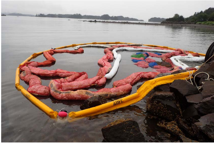
Aggressive booming of the storm drain outfall during the Jarvis Power Plant diesel release, August 2015 (Photo/DEC- Bob Mattson)
