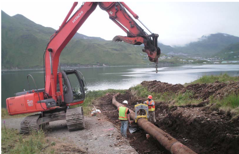
Cutting and removal of pipeline 214 (Photo/ Bristol Environmental Remediation Services, LLC.)
