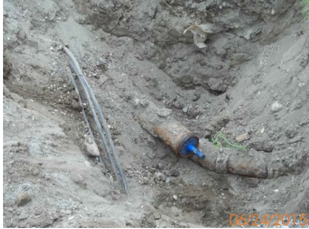
900-gallon UST excavation at former dry cleaner (left), sewer line excavated, cut, and plugged at former dry cleaner, June 24, 2015 (Photo/DEC)
