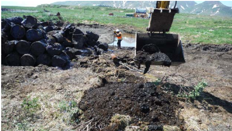
Excavation of drums and contaminated soil at AO#1 (Photo Bristol Environmental)
