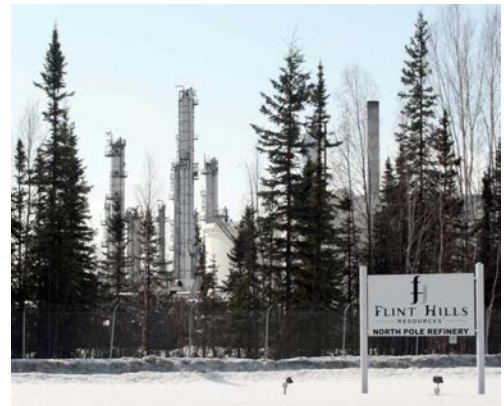
Flint Hills Refinery in North Pole (Photo/DEC)
