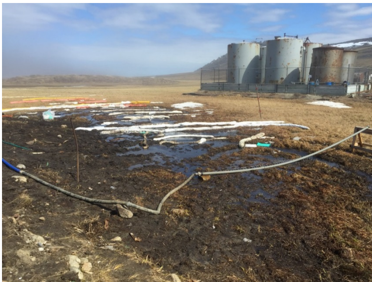
Flush and recovery tactic implemented behind the clinic building. The grey hose in the foreground supplied water while the absorbent materials captured the mobile hydrocarbons brought up by the water deluge tactic, June 11, 2016 (Photo/DEC- Kelley Tu)
