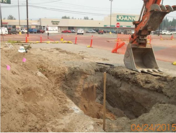
900-gallon UST excavation at former dry cleaner (left), sewer line excavated, cut, and plugged at former dry cleaner, June 24, 2015 (Photo/DEC)
