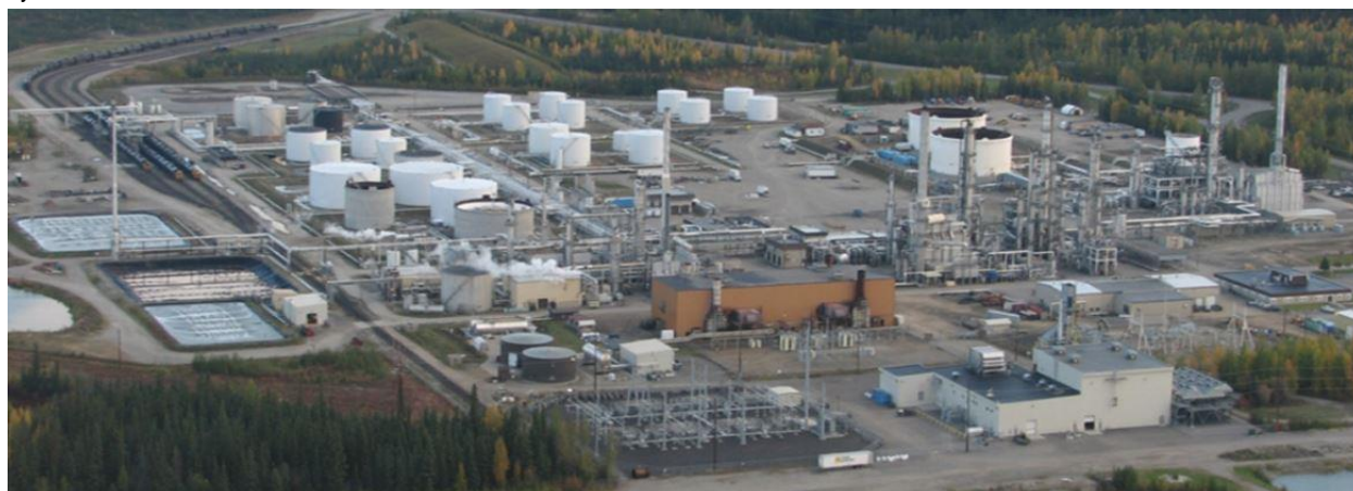
Aerial view of Flint Hills Resources' North Pole refinery from the south. (Photo/Flint Hills Resources)
