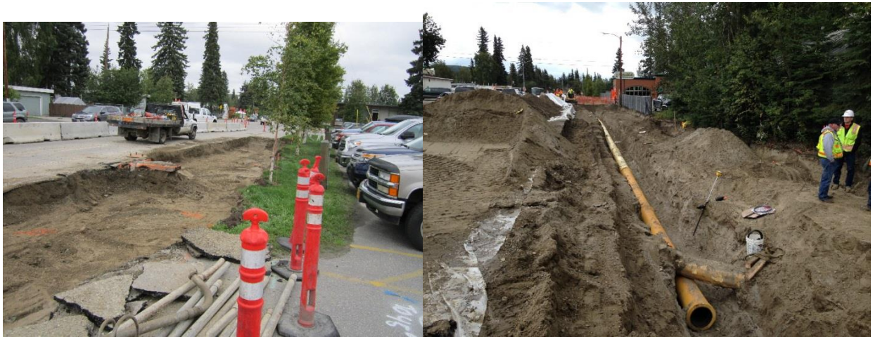
College Road Reconstruction, Fairbanks, June 2015 (Photo/DEC)
