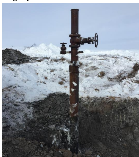
Umiat Test Well #10 excavated for removal of the wellhead. (Photo/BLM-Robert Brumbaugh)
