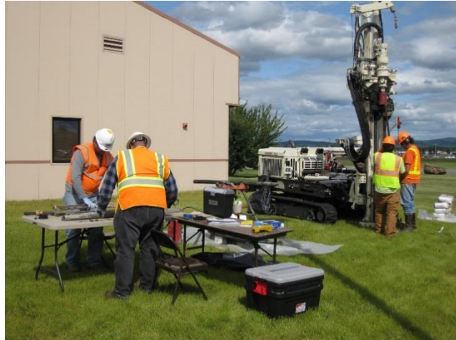
Site work underway on Eielson AFB
