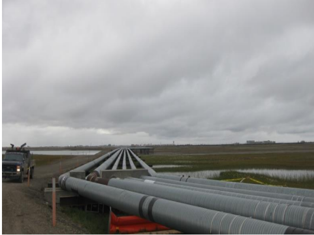
180 miles of flow lines were inspected in FY15 (Photo/DEC)
