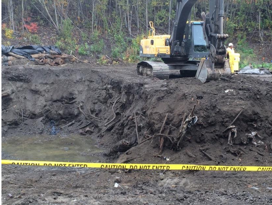
Time Critical Removal Action at Galena former AFS. Phase 1(Photo/DEC)
