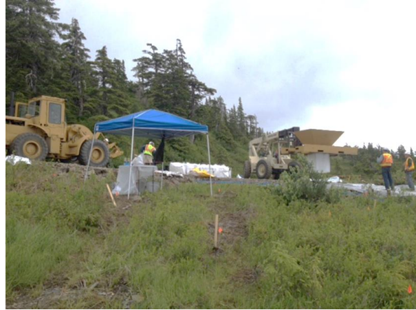
Duncan Canal work site. (Photo/DEC- Anne Marie Palmieri)
