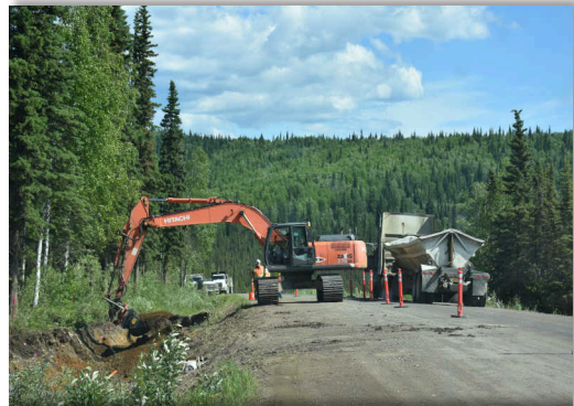
Dalton Highway Truck Rollover, contaminated soil being loaded into a dump truck for disposal June 14, 2019 (Photo/ DEC)
