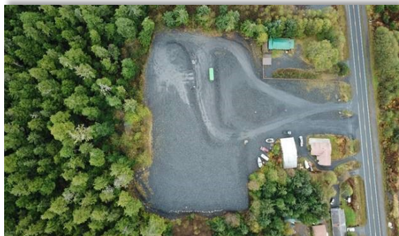
Final site conditions at Wrangell Junkyard in October 2018. (Photo/NRC Alaska)
