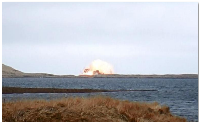
Navy Explosive Ordnance Disposal staff open the Andrew Lake Spillway each year with explosives as a means to control lake water levels and ensure the contractors have access to the Remedial Action Areas, 2014 (Photo/U.S. Navy)
