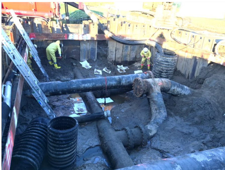
Excavation activity at dig site 1, September 23, 2016 (Photo/DEC)
