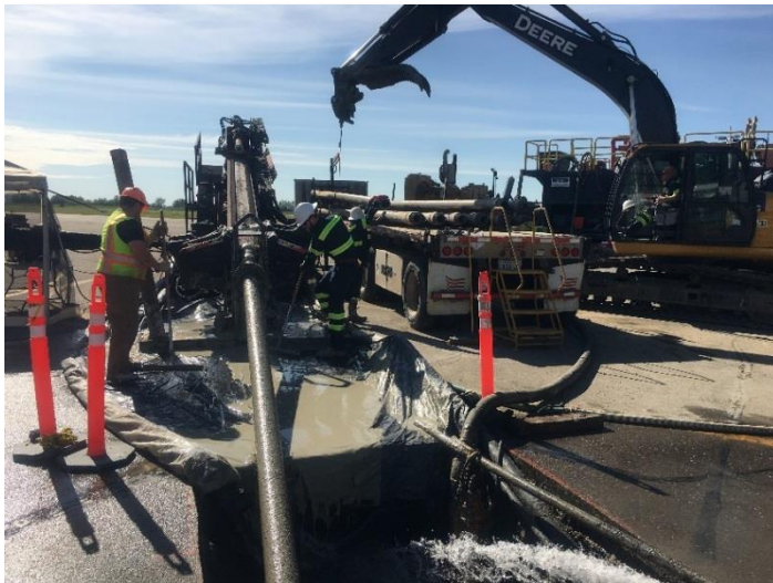
Horizontal drilling and sparge well installation at Galena, 2017 (Photo/DEC)
