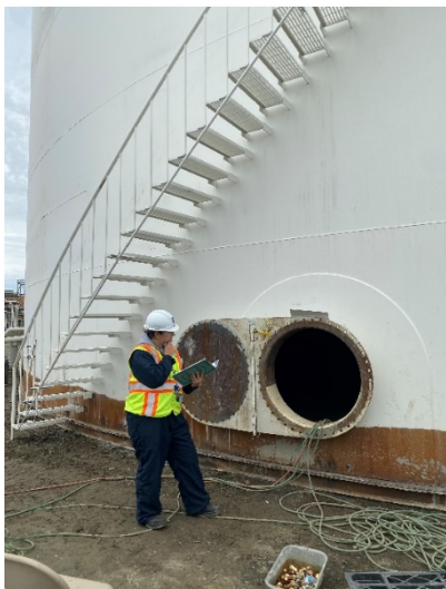
SPAR staff conduct terminal tank farm inspections at the North Pole facility in 2020. (Photo/DEC)
