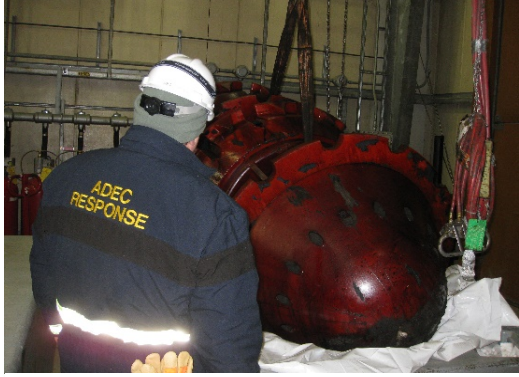
A SPAR responder at a pipeline cleaning shutdown in February 2011. The device pictured, known as a pig, is used to clean and track critical maintenance for oil transport pipelines. (Photo/DEC)
