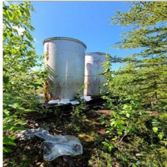
Home heating oil fuel tanks near Shungnak School along the Kobuk River on June 22, 2020. (Photo/DEC)
