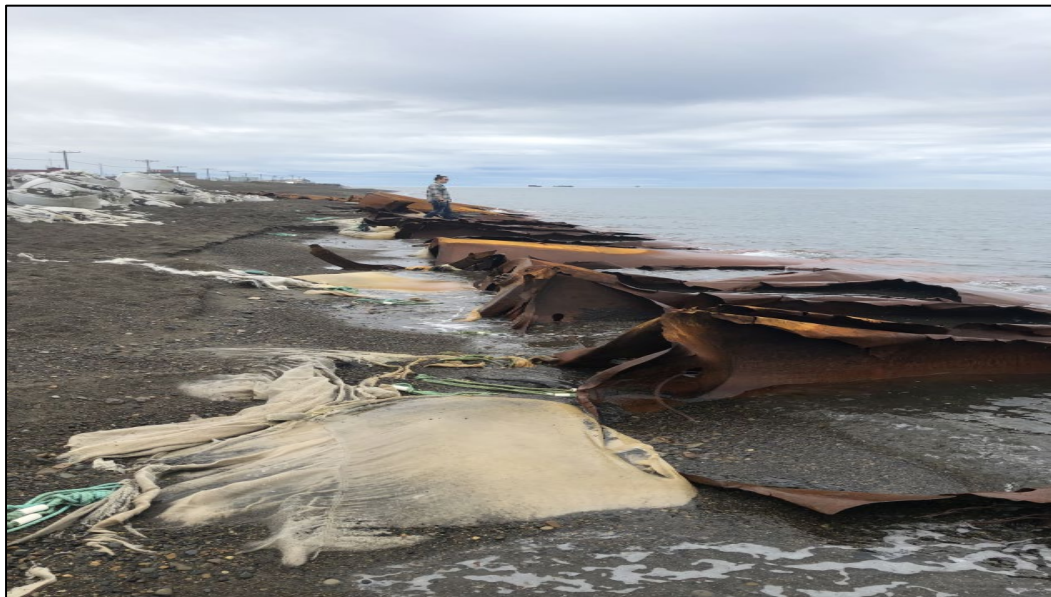
Old drums used for erosion control on the coast. Photo Credit: North Slope Borough (Robert Sceeles)
