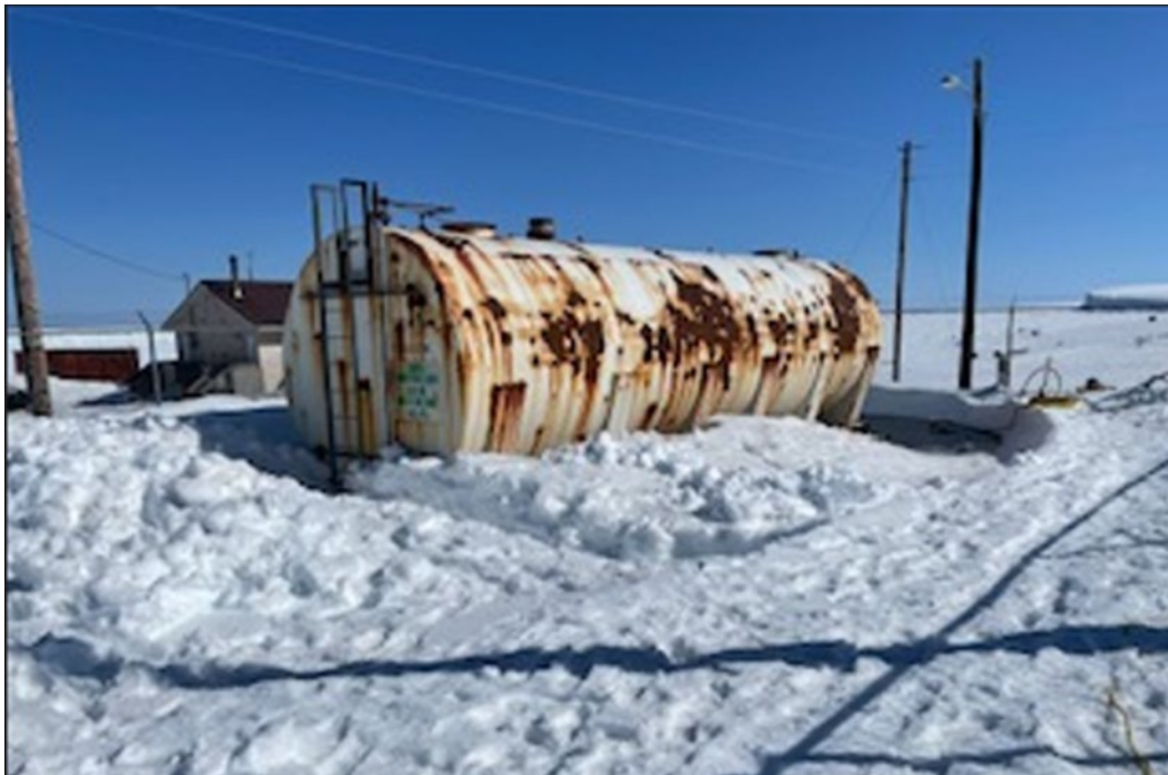
27,000 gallon diesel tank that leaked into secondary containment. Fuel can be observed pooled to the right of the tank.
