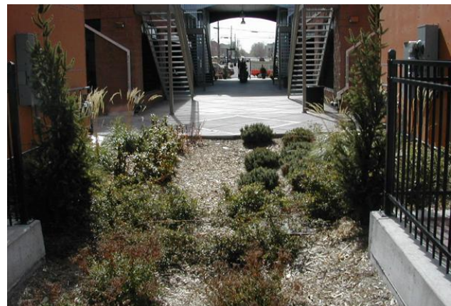
EXHIBIT 6.68 POROUS LANDSCAPE DETENTION IN DENVER
