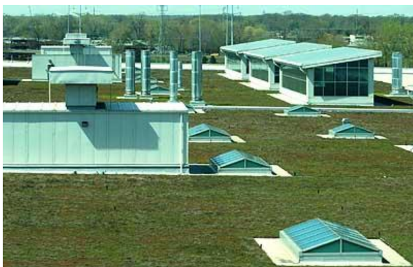
EXHIBIT 6.30 INDUSTRIAL FACILITY “LIVING ROOF” IN DEARBORN, MI
