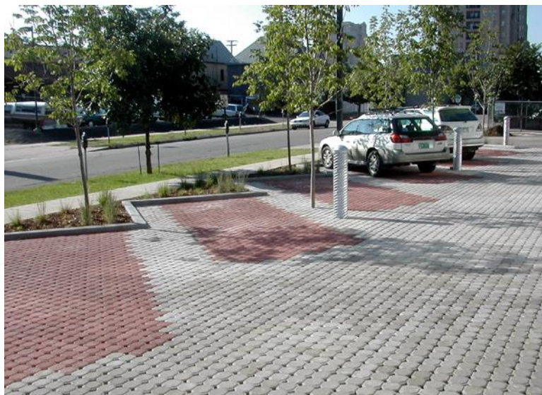
EXHIBIT 6.63 COBBLESTONE BLOCK POROUS PAVEMENT IN DENVER
