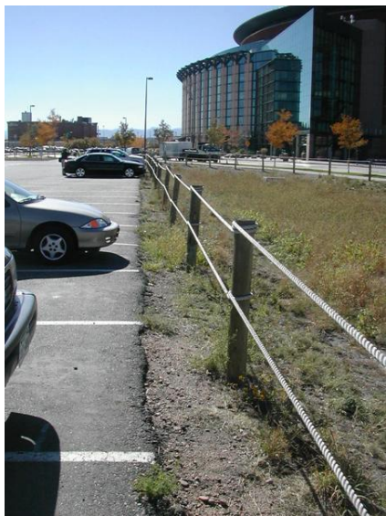
EXHIBIT 6.73 EXTENDED DETENTION BASIN AT SPORTS ARENA IN DENVER
