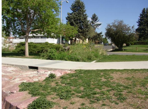
EXHIBIT 6.67 POROUS LANDSCAPE DETENTION IN DENVER
