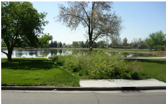
EXHIBIT 6.24 POROUS LANDSCAPE DETENTION AT HUSTON LAKE PARK IN SOUTHEAST DENVER
