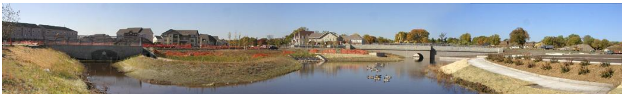
EXHIBIT 6.22 WET POND IN NEIGHBORHOOD PARK IN MINNEAPOLIS, MN
