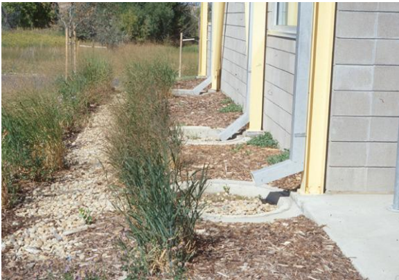
EXHIBIT 6.28 DOWNSPOUTS IN BOULDER
