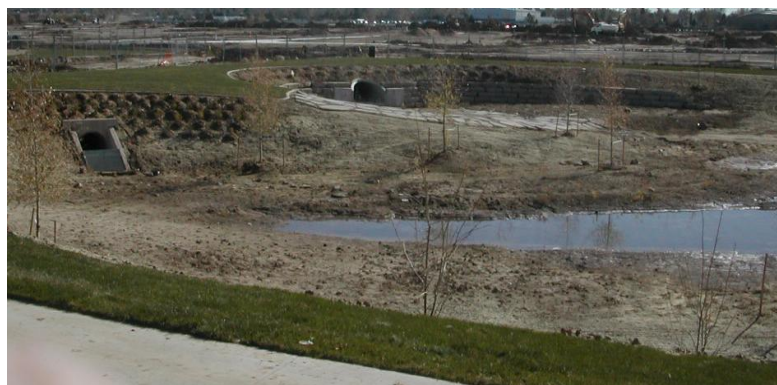
EXHIBIT 2.5 RECENTLY CONSTRUCTED DETENTION BASIN (VEGETATION NOT YET ESTABLISHED) ON WESTERLY CREEK IN THE STAPLETON REDEVELOPMENT AREA
