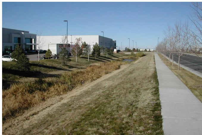
EXHIBIT 6.16 LINEAR DETENTION POND AT AN INDUSTRIAL SITE
