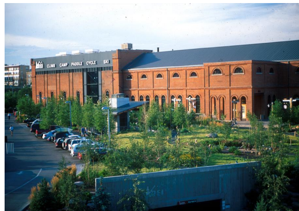
EXHIBIT 6.11 GREEN ROOF PARKING STRUCTURE IN DENVER
