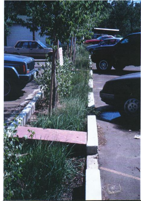
EXHIBIT 6.34 PARKING MEDIAN POROUS LANDSCAPE DETENTION IN BOULDER
