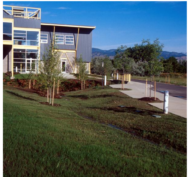
EXHIBIT 6.59 GRASS SWALE IN BOULDER
