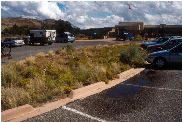
EXHIBIT 6.36 SLOTTED CURB IN CANYONLANDS NATIONAL PARK, UT
