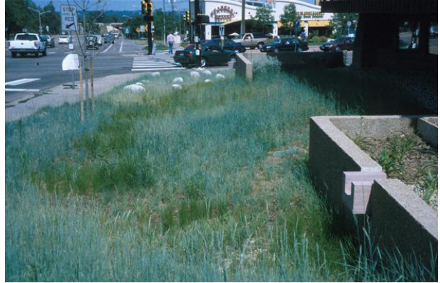
EXHIBIT 6.57 GRASS SWALE IN BOULDER
