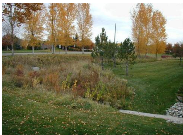
EXHIBIT 6.47 DETENTION BASIN WETLAND MICROPOOL IN AURORA
