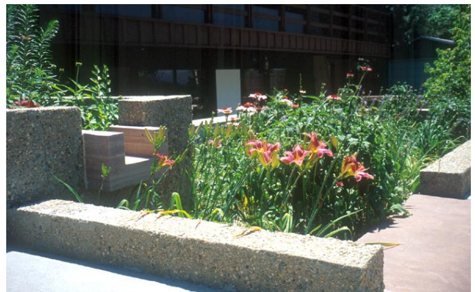
These planter boxes fill with water, infiltrating significant amounts of stormwater before overflowing into treatment areas, while appearing beautiful throughout the year.
