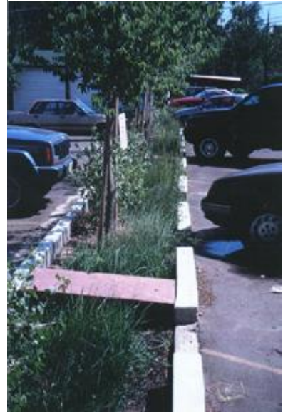
This linear treatment area between two bays of parking takes advantage of the landscape strip to infiltrate stormwater.
