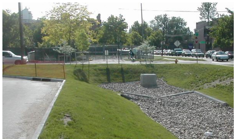
EXHIBIT 6.74 EXTENDED DETENTION BASIN IN DENVER
