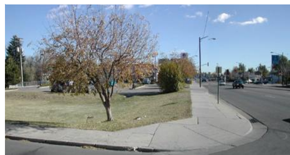
EXHIBIT 6.5 DETENTION BASIN IN DENVER
