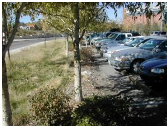
Between the parking lot and the street, this swale creates a landscape buffer between two paved areas
