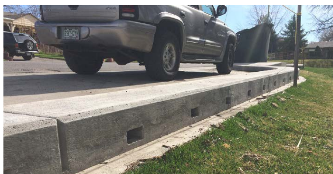
FIGURE 5. Back side of forebay (Source: UCFCO. 2015)
