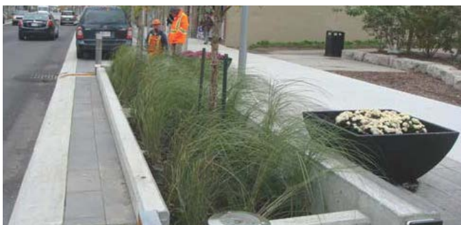
FIGURE 2. Example of stormwater planter
