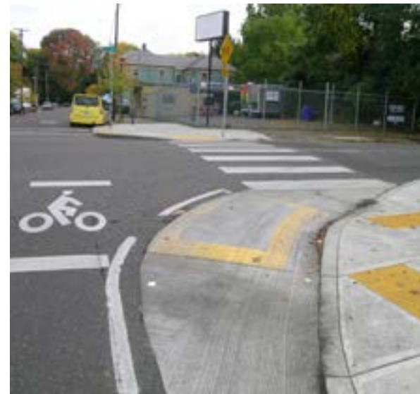
Truck aprons offer tighter turning radii for passenger vehicles while still allowing large trucks to mount the apron and maneuver through turns. The photo at left is a truck apron in Portland, OR.
