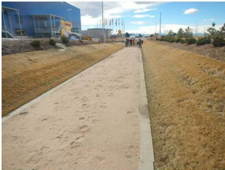
Clean Sand Filter media No immediate maintenance required
