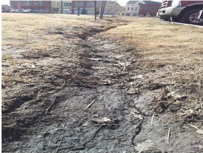
Swale bottom has erosion and excessive sediment build-up Maintenance required
