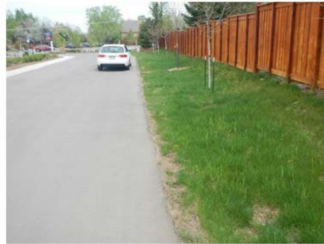
Grass Swale with reasonable vegetation and no major issues No immediate maintenance required
