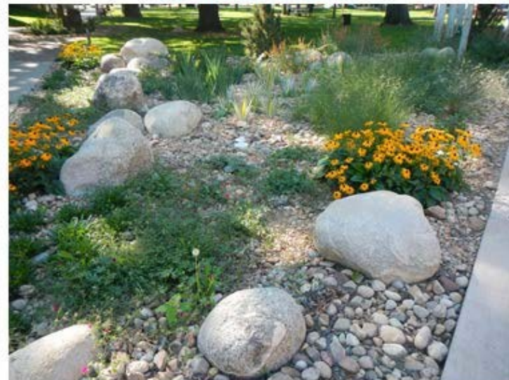
Rain Garden with healthy vegetation No immediate maintenance required
