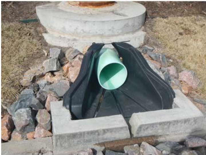
Clean forebay No immediate maintenance required
