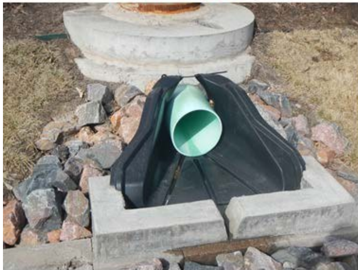
Clean forebay No immediate maintenance required
