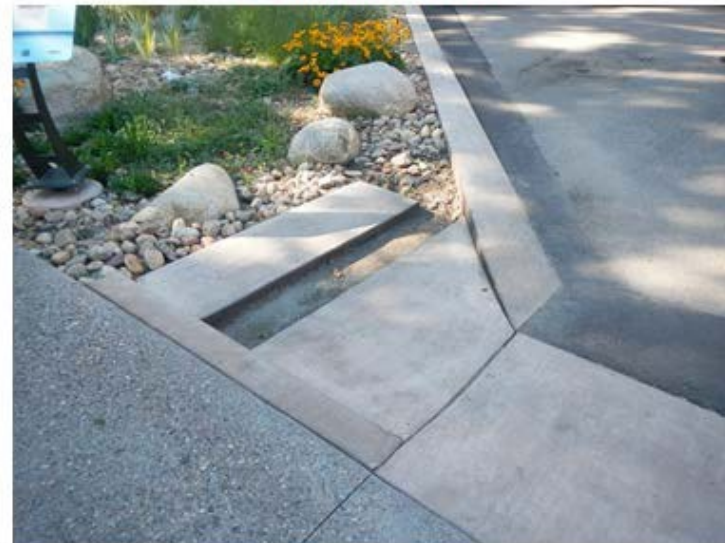
Clean forebay No immediate maintenance required
