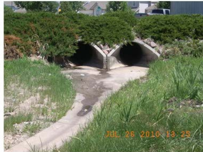
Clear inlet with no major issues No immediate maintenance required
