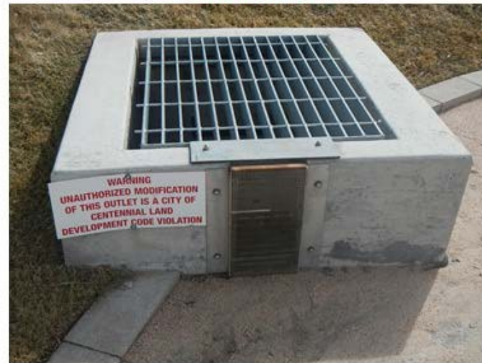
Outlet Structure in good condition No immediate maintenance required
