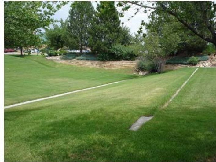
Basin area has healthy turfgrass No immediate maintenance required
