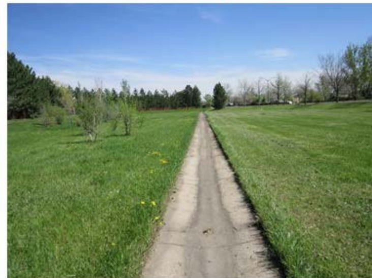
Clear trickle channel No immediate maintenance required
