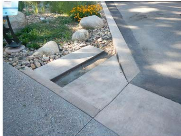
Clean forebay No immediate maintenance required
