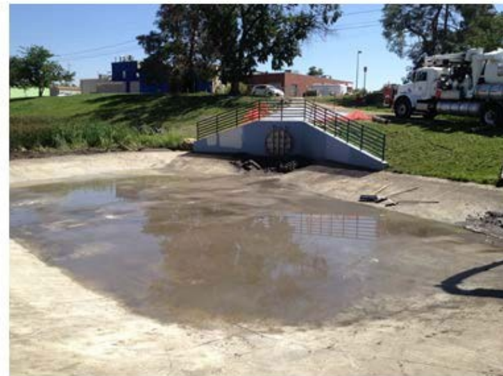
Clean, dry forebay with limited sediment accumulation No immediate maintenance required
