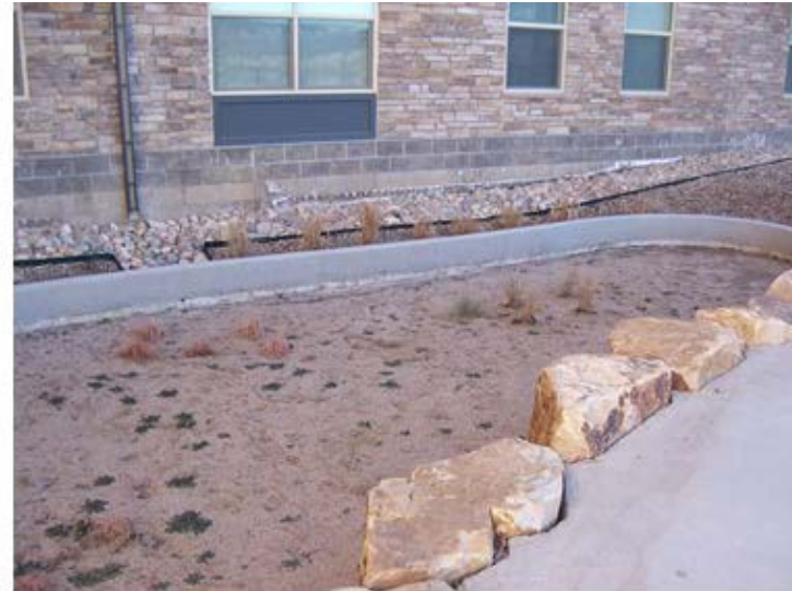
Sparse vegetation in rain garden Maintenance required
