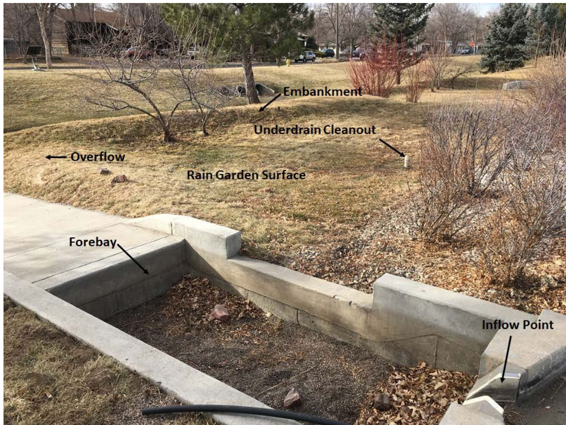
Figure 5. Typical Rain Garden Features
