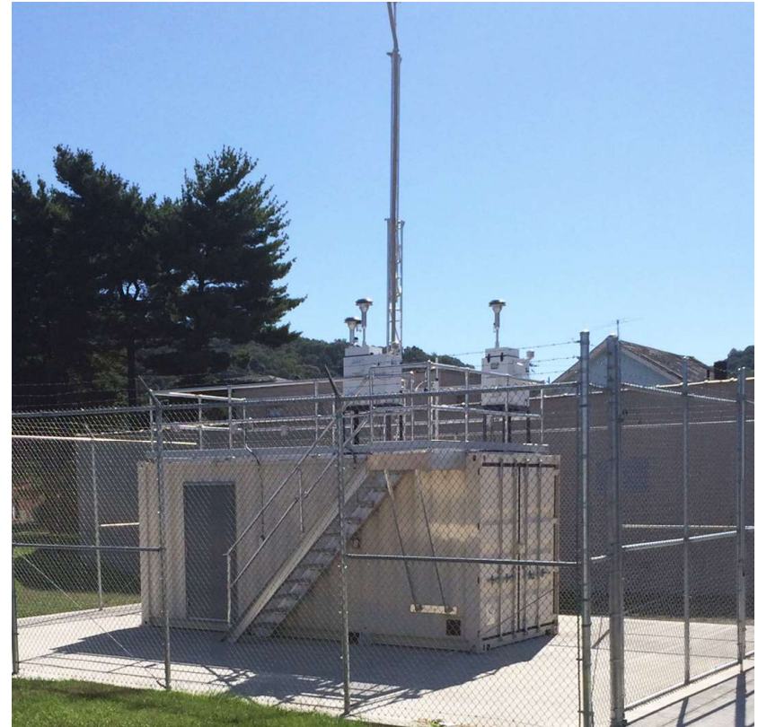
NCore site located in Charleston, West Virginia
