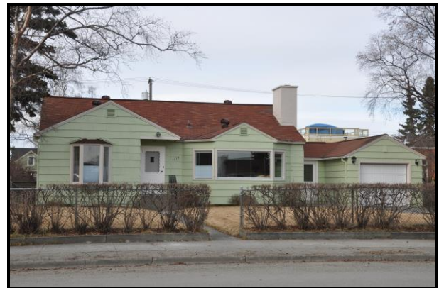
Residential Building, South Addition, Anchorage
