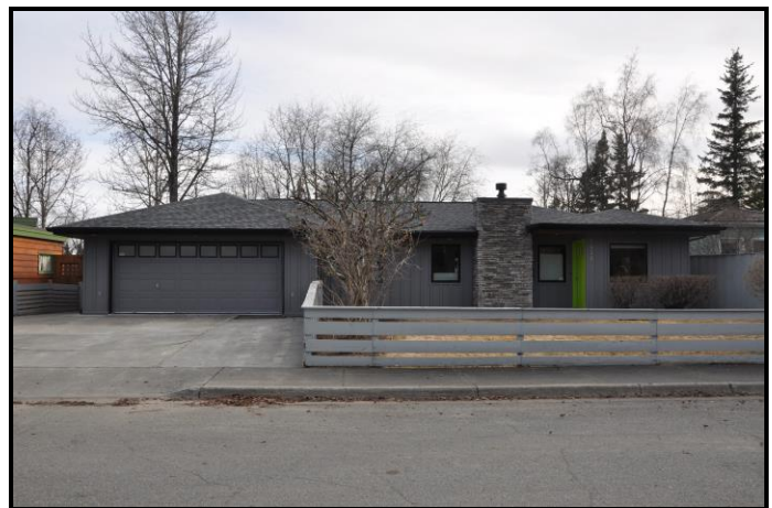
Residential Building, South Addition, Anchorage
