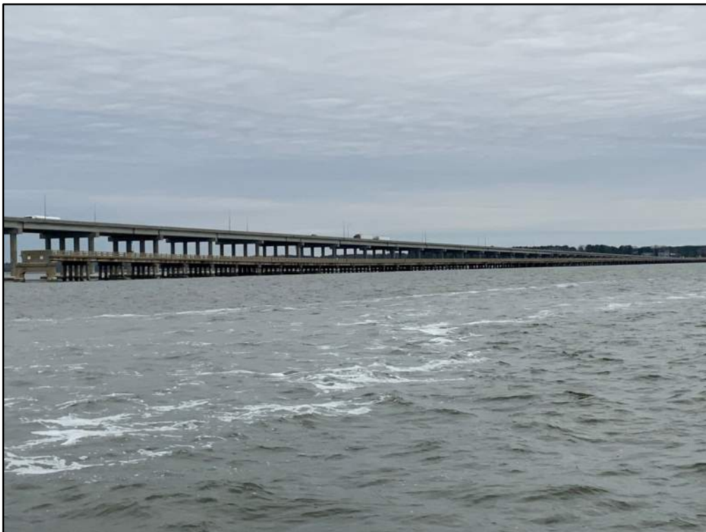
Photo 2: Overall of the North Half of the Pier (East Elevation).
