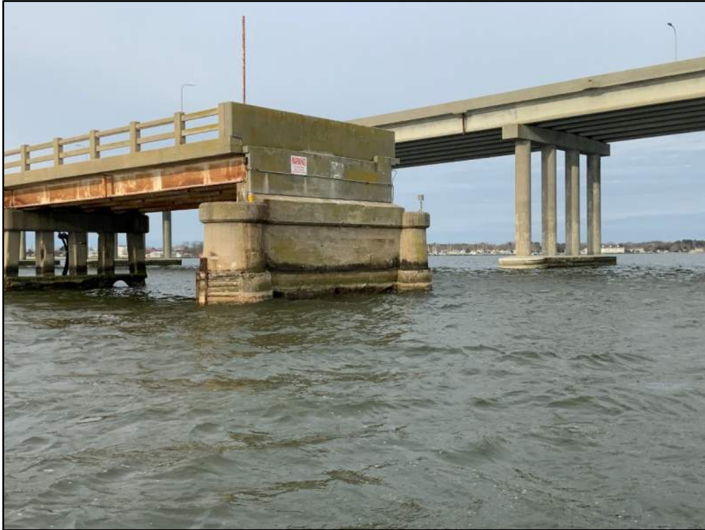
Photo 7: South Elevation of Pier Wall 1 (Bent 56).
