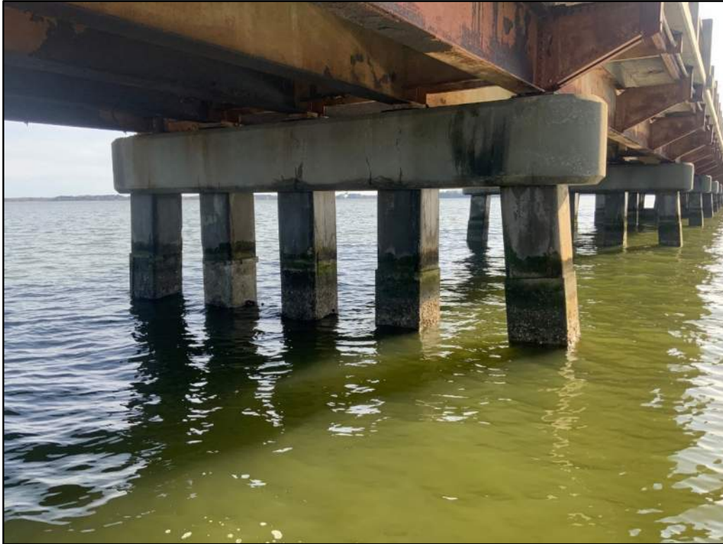
Photo 5: Typical Bent without a Reinforced Concrete Strut (Bent 129 Shown).
