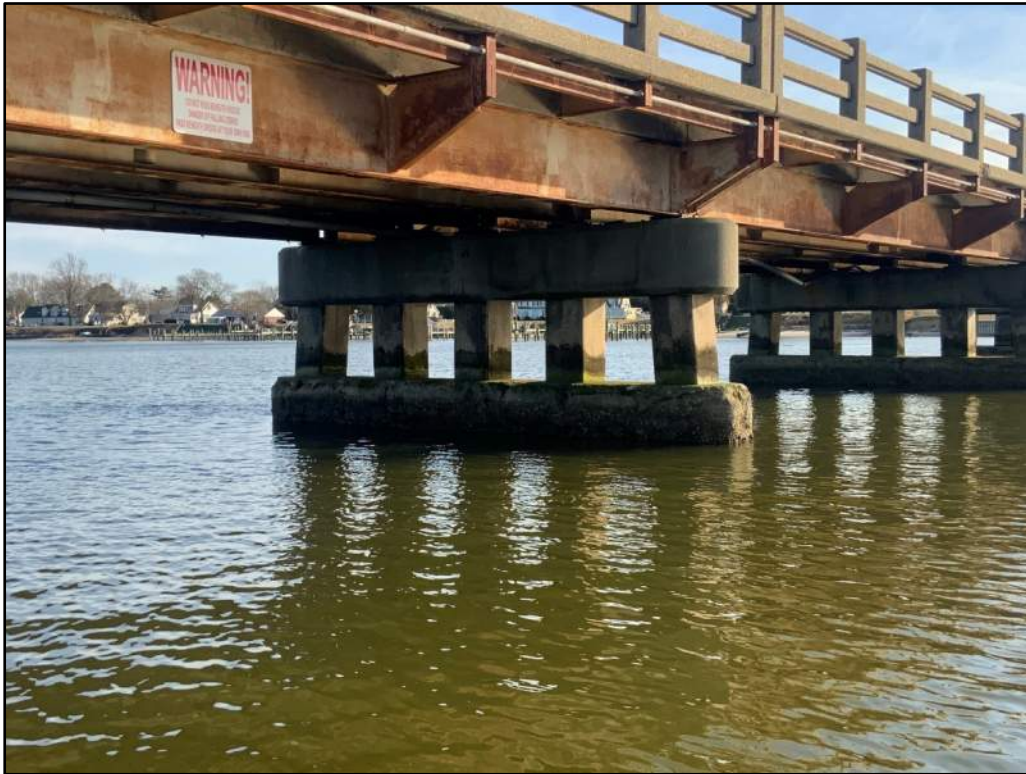
Photo 3: Typical 5-Pile Bent (Bent 8, North Elevation Shown).
