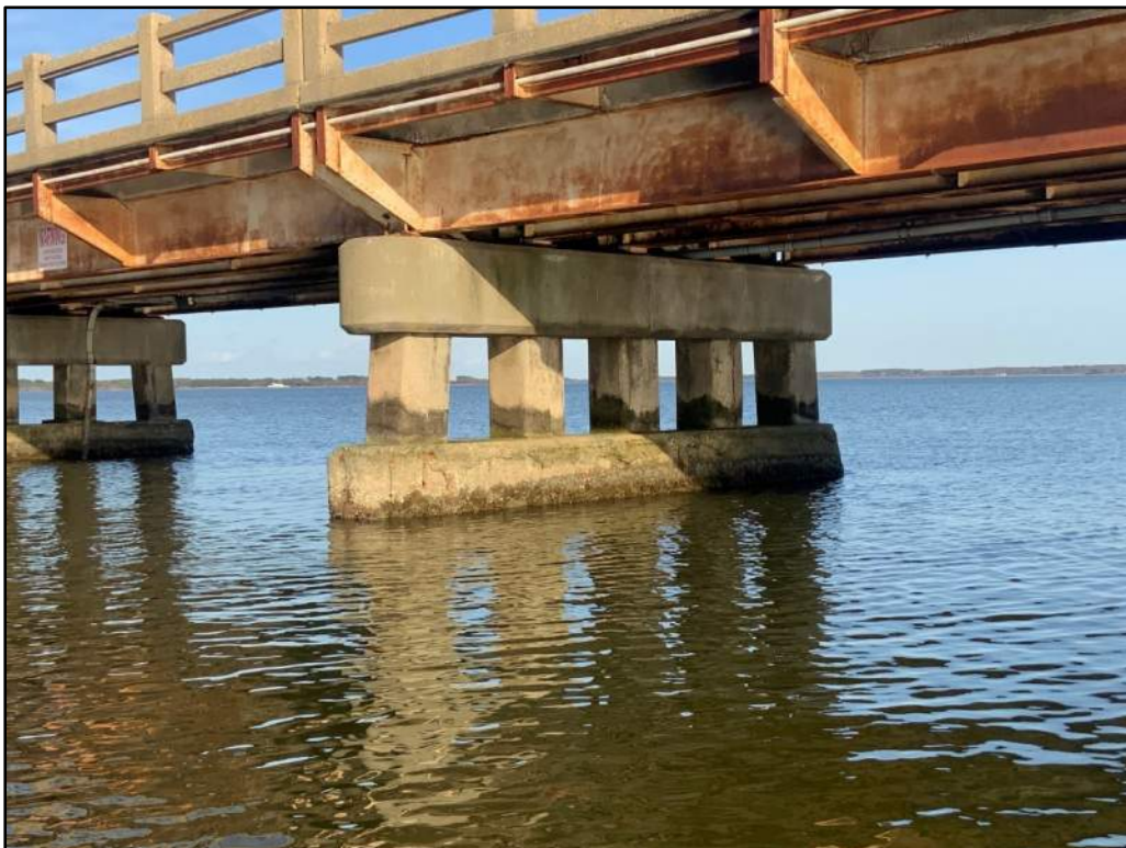
Photo 4: Typical 5-Pile Bent (Bent 10, South Elevation Shown).
