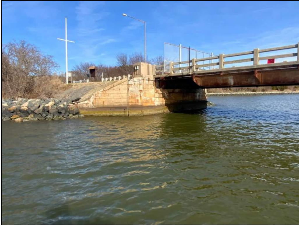
Photo 9: North Abutment Elevation Looking Northeast.
