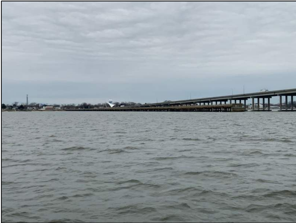
Photo 1: Overall of the South Half of the Pier (East Elevation).
