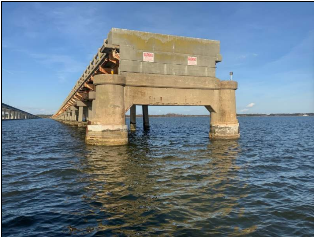
Photo 8: North Elevation of Pier Wall 6 (Bent 57).
