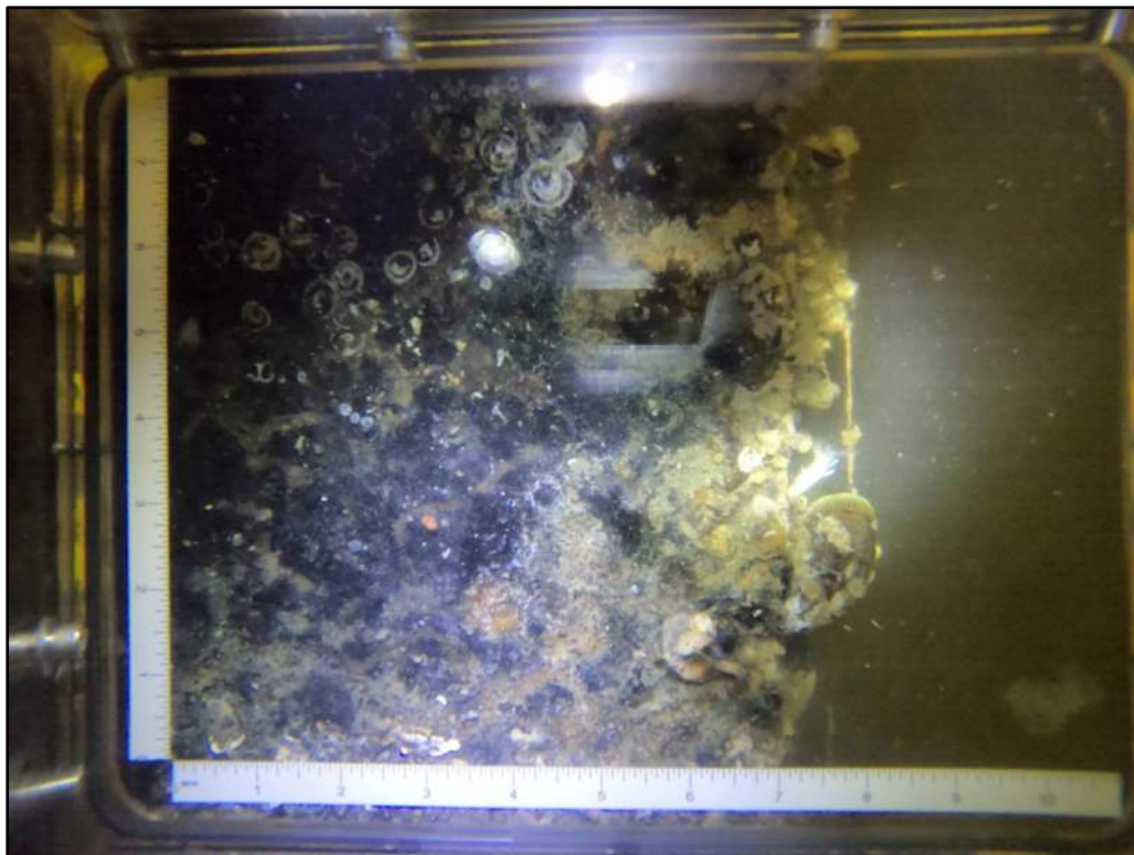
Photo 30: Pier Wall 6 (Bent 57), Typical Condition of Footing (Underwater).
