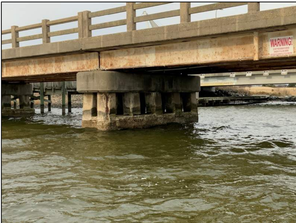
Photo 6: Typical 10-Pile Double Bent (Bent 8, North Elevation Shown).
