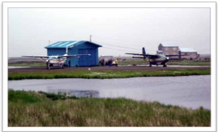
Kwigillingok Airport Most rural airports consist of a runway, apron, access road and snow removal building. FAA funded $1.5 million in 2011, for much needed runway repairs at this airport.
