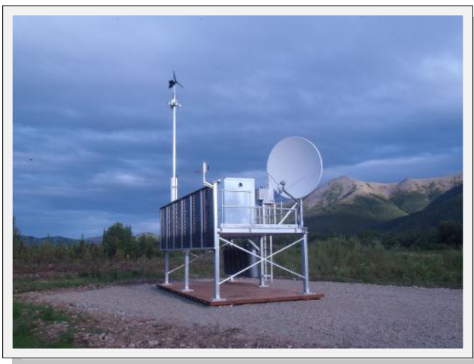
(L-R) Remote solar/wind platform supports cameras at the Nycac Airport and Lake Clark East.
