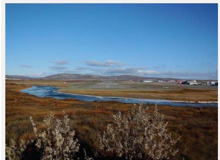
Nome Airport - new runway safety area constructed on Runway 3. DOT&PF Project Photo
