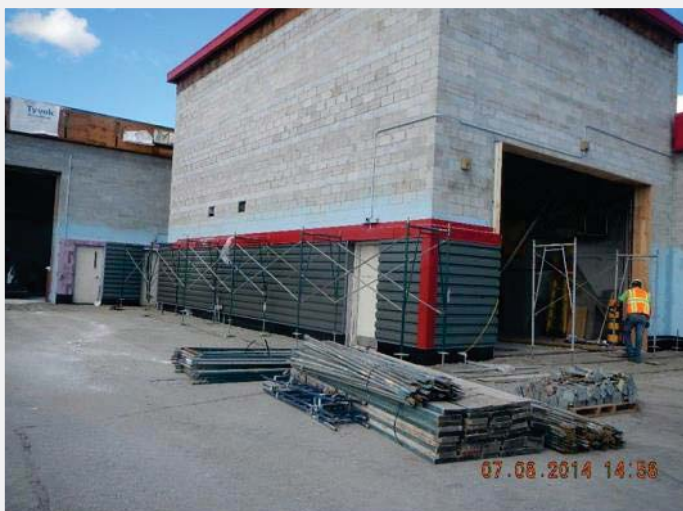
ARFF building at FAI was rehabilitated in 2014
