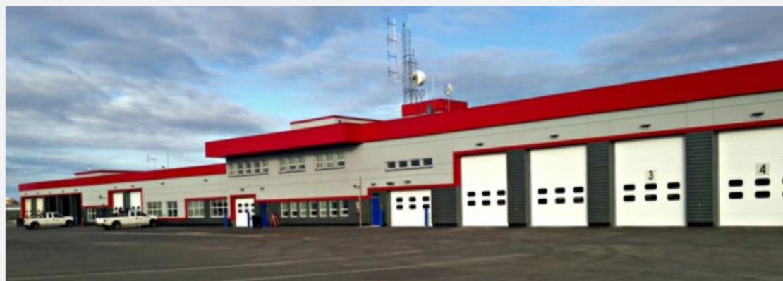
The newly remodeled Fairbanks Airport Response Center houses Airport Police and Fire, Dispatch, Badging, Field Maintenance, and Operations.
