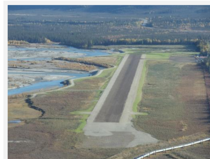
Coldfoot Airport was resurfaced in 2016
