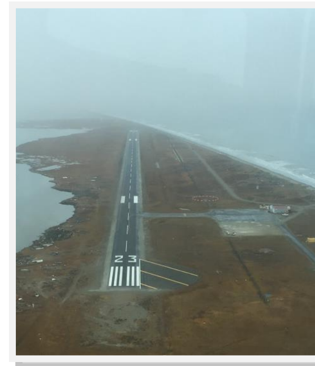
Newly resurfaced Shishmaref Airport
