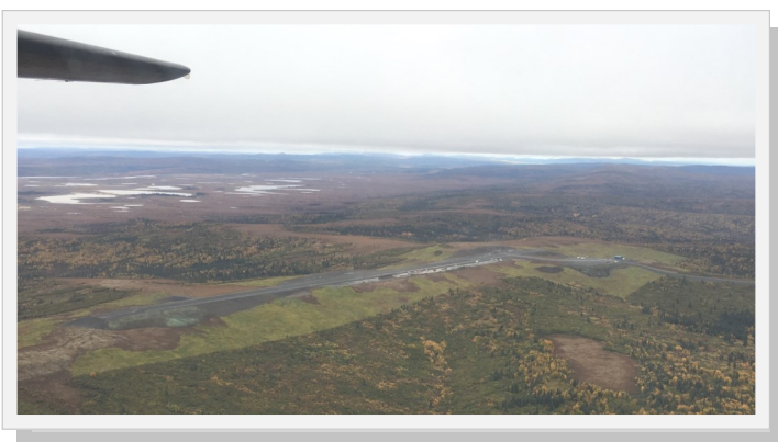
The new Pilot Station Airport Runway
