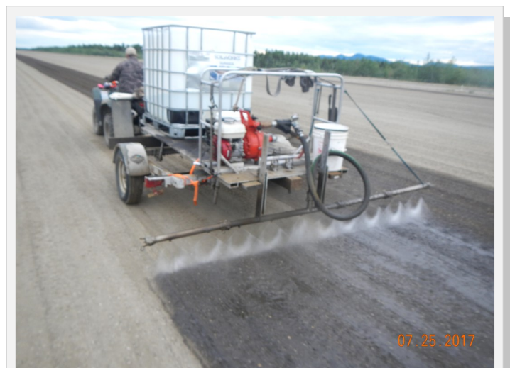
Photo - example of surface preservation maintenance at Bettles Airport
