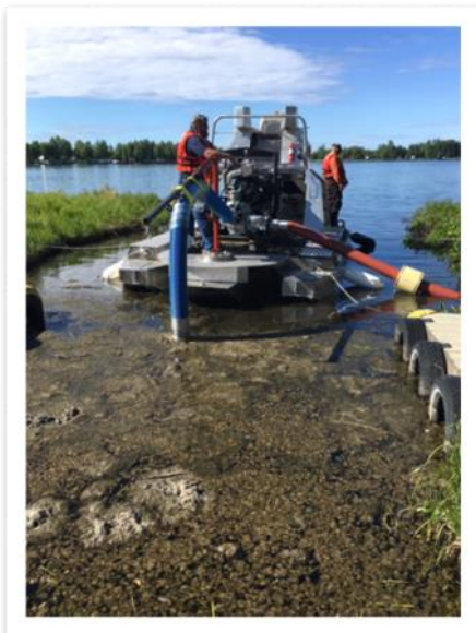
The Work Barge
