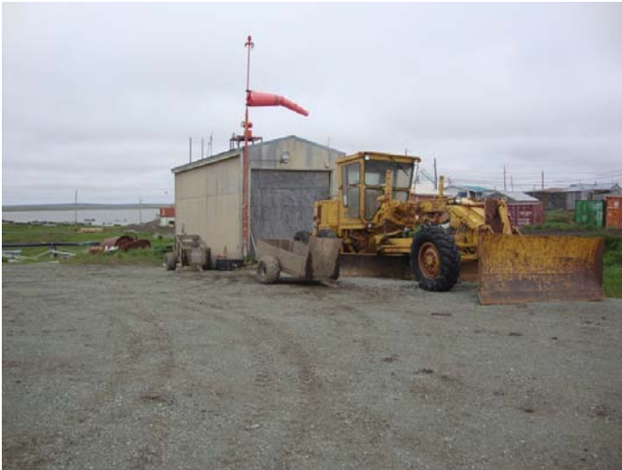
Kipnuk's snow removal equipment building and grader.
