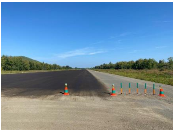
Holy Cross Airport project included installing surfacing, dust palliative, lighting systems, and FAA Nav aids. The final inspection occurred in August and the project is almost complete.
