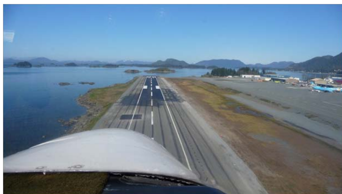
First night's work completed. (Photo courtesy - Chuck Tripp, DOT&PF)
