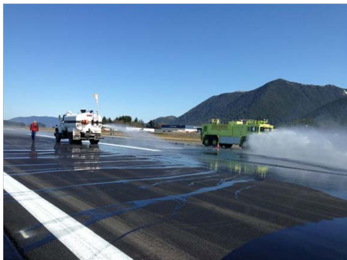
Preparing for morning reopening. (Photo courtesy - Maureen Hanson, DOT&PF)
