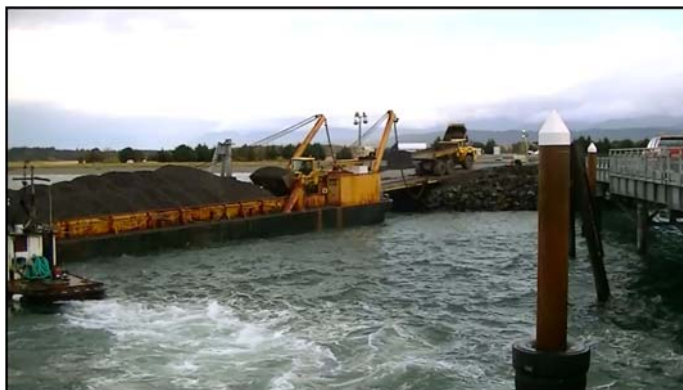
Gravel being offloaded from a barge for the Gustavus Airport.
