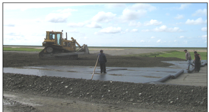
Placement of geotextile separation and sub base at the Alakanuk Airport.
