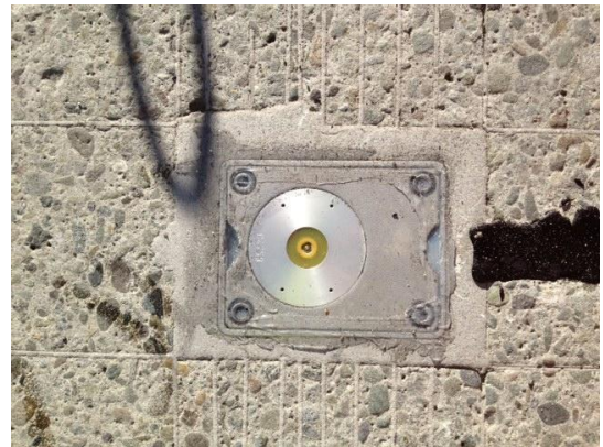
Temperature Sensor in the Knik River Bridge Deck Steve Banse, ADOT&PF
