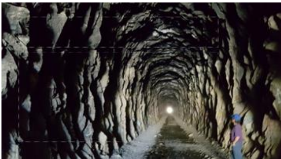
Image of the “Summit Tunnel”, part of the Transcontinental Railway and one of seven sites that traverses Auburn, CA to Donner Pass.
