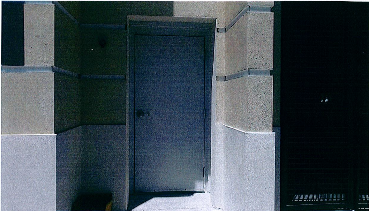
Stair #3 door alteration.
