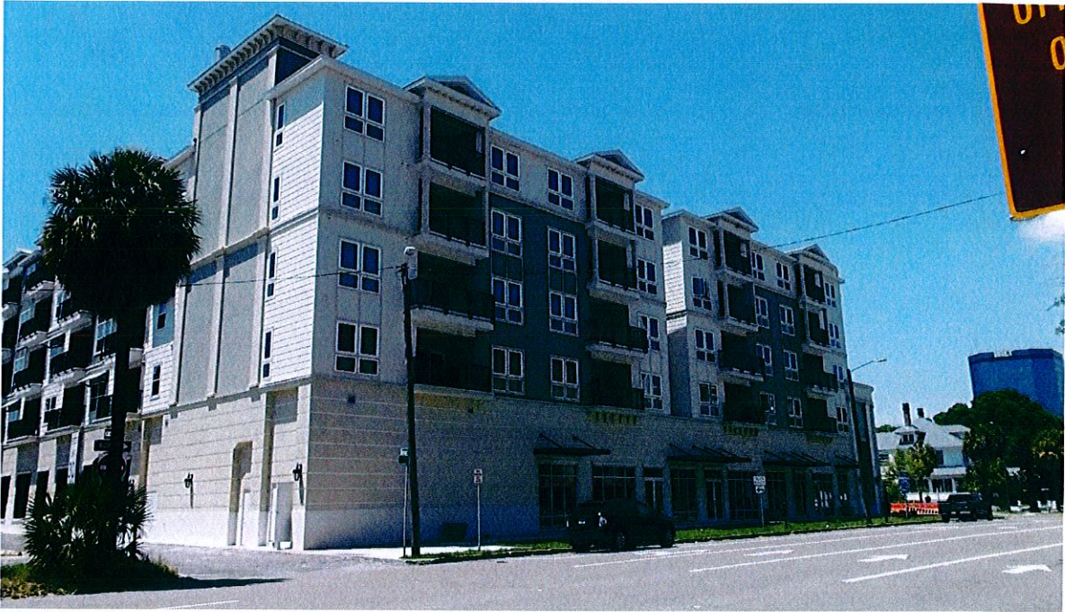
3 rd St S and Delmar Terrace.
