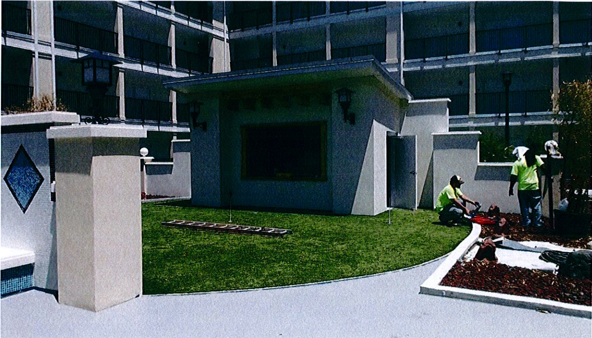
Courtyard bench seat and traction coating.
