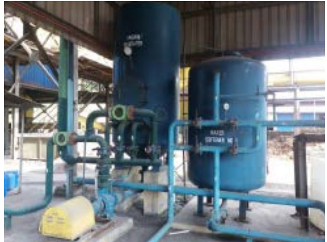
Water transfer pump (SIHI model ULNC)
