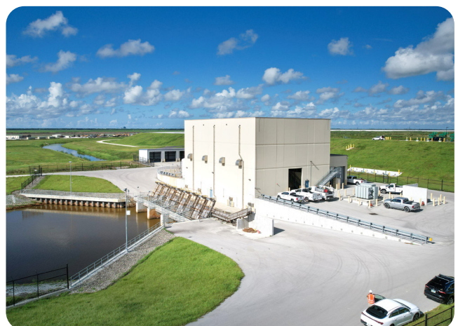
C-44 S-401 pumping station
