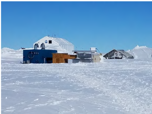
View of SMG and Microturbine and SOB demolition activities.
