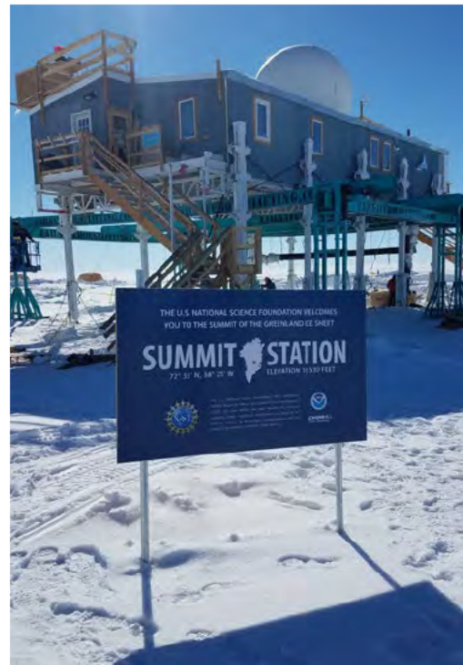
Summit Sign and Big House. Note the lifting system being used.
