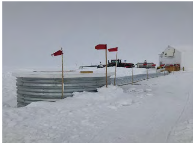
Photo of SMG Vault and Utility Corridor
