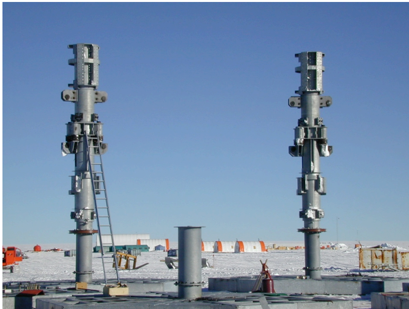
Figure 19. Constructing the lifting columns on site (courtesy of P. Godon 2010).
