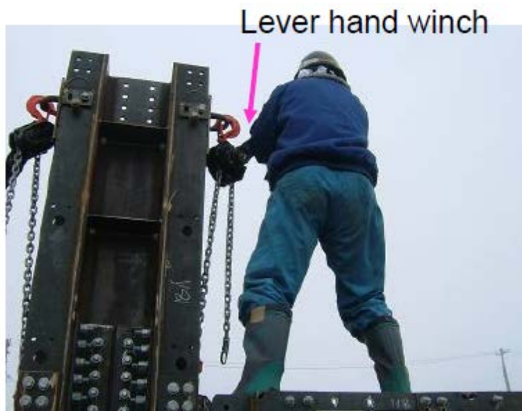
Figure 22. Lever hand winch is the lifting mechanism to raise the structure (courtesy of K. Ishizawa, Japan NIPR).
