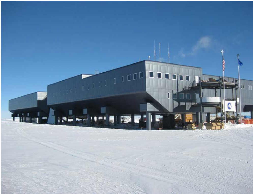
Figure 20. The Amundsen-Scott South Pole Station supports the U.S. Antarctic Program.
