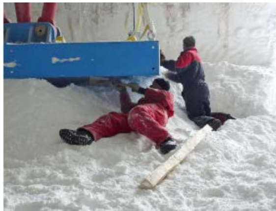
Figure 13. Back-filling snow under a raised footpad (Rotthäuser and Jagolski 2010).
