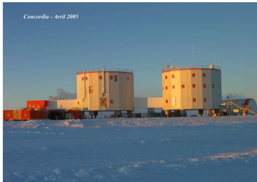
Figure 17. Completed Concordia Station, April 2005. The three buildings from left to right are the power plant and mechanical systems, the “Noisy” building, and the “Quiet” building (courtesy of P. Godon).
