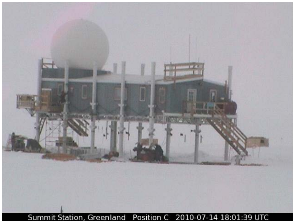
Figure 7. Summit Station's “Big House” after it was lifted 4.5 m in 2010.
