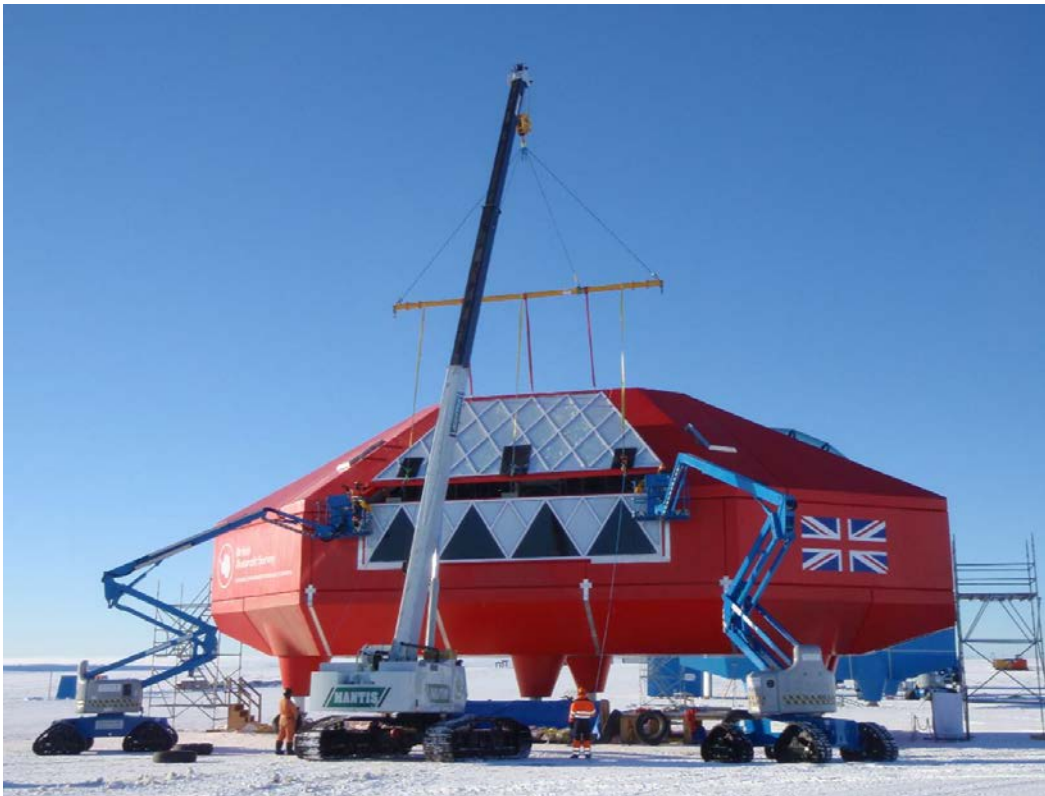
Figure 14. Construction of Halley VI's central living module (Broughton 2010).
