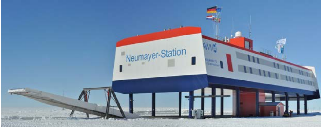
Figure 9. The commissioned Neumayer III Station. Note the raised roof of the ramp in the left of the photo, which leads down to the subsurface garage and storage area directly below the elevated building. The roof is lowered during storms (Gernandt et al. 2010).
