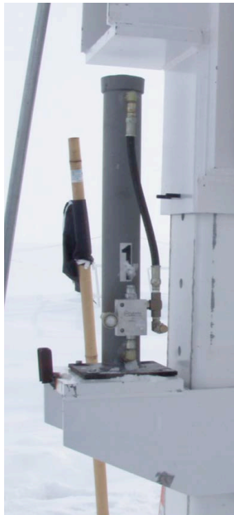
Figure 8. Position of the hydraulic jack used for the “Big House” lift procedure (Barna et. al. 2011).
