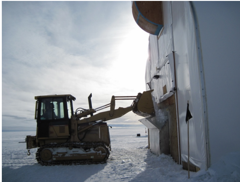
Figure 1. Caterpillar 933, used for snow mining at Summit Station, dumping snow into the chute leading to the melt tank.
