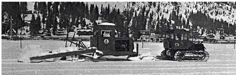
Figure A4. Navy Model 42 Snow Pulvimixer being towed by a tractor (Camm 1961).
