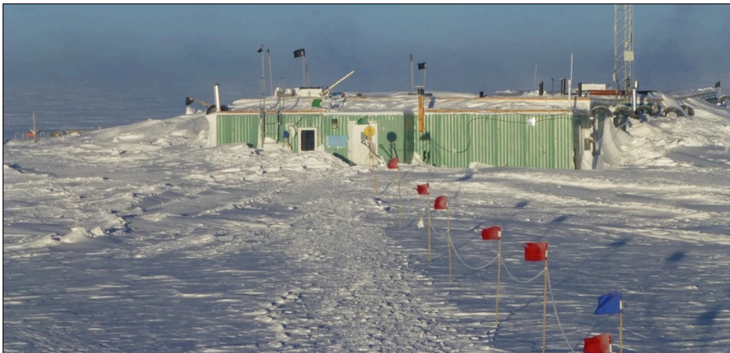
Figure 1. Drifting snow around the Green House, February 2015. (Photo courtesy of Polar Field Services, Littleton, CO.)
