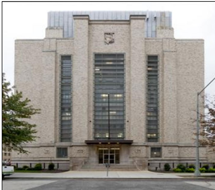
Figure 1. Central Heating Plant, Washington D.C. 1
