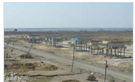
Figure 3 An aerial view of nine of the 10 Fortified homes still standing following Hurricane Ike amid the rubble of other traditionally built houses that did not survive.
