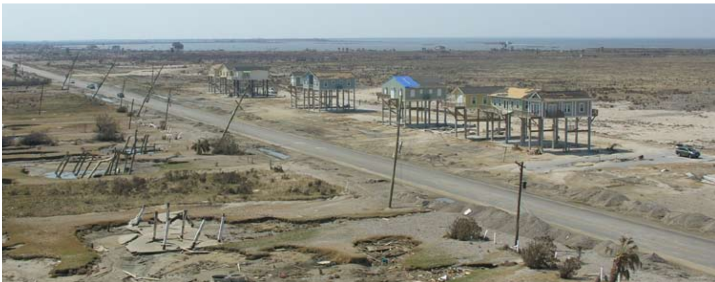
Fortified homes that survived Hurricane Ike on the Bolivar Peninsula, Texas.
