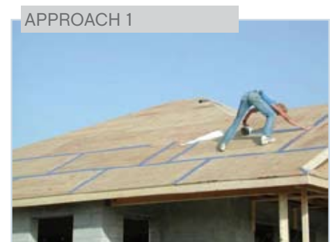
Zones where close spacing of fasteners is most critical during re-nailing of sheathing.
