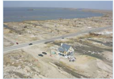
Figure 15 This home was dubbed the “Last House Standing” by the media, but did not perform as well as the houses built to the IBHS Fortified...for safer living® standard.
