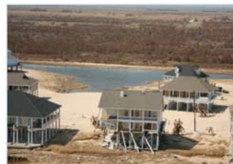
Figure 20 A number of houses near the coast clearly had piles that continued through the height of the first floor. In these houses, the upper floors appeared to remain intact, but frequently the bottom floor and parts of the walls on the bottom floor were completely missing.
