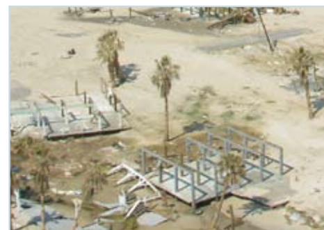
Figure 19 Houses near the Gulf of Mexico where the piles terminated at the bottom of the first floor tended to be completely wiped out by the storm surge.
