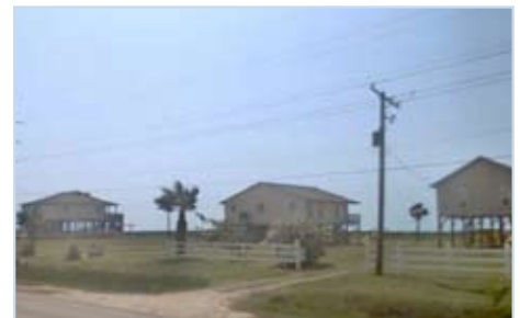
Figure 2 Older traditionally built homes before Hurricane Ike. These houses, located directly south of some of the Fortified homes in Figure 4, were on the narrow strip of land on the Gulf side of the highway before being destroyed by Ike.
