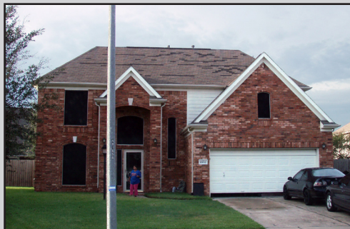
WIND UPLIFT OF INDIVIDUAL TABS AND SHINGLES
