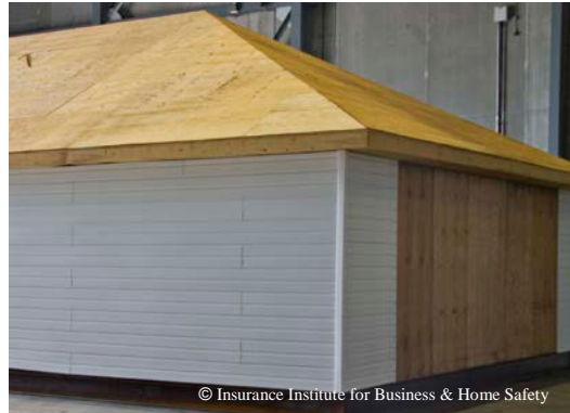
Figure 6: Cornering Detail on Vinyl Siding
