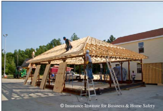
Figure 5: Construction of Gable/Hip Test Building with 6-on-12 Pitch Roof
