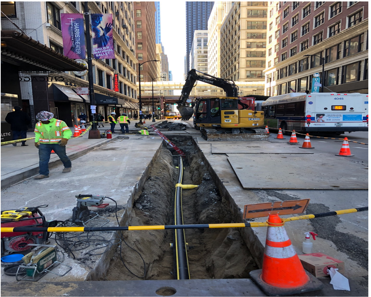
Gas main being installed in Madison Ave. near Michigan Ave.
