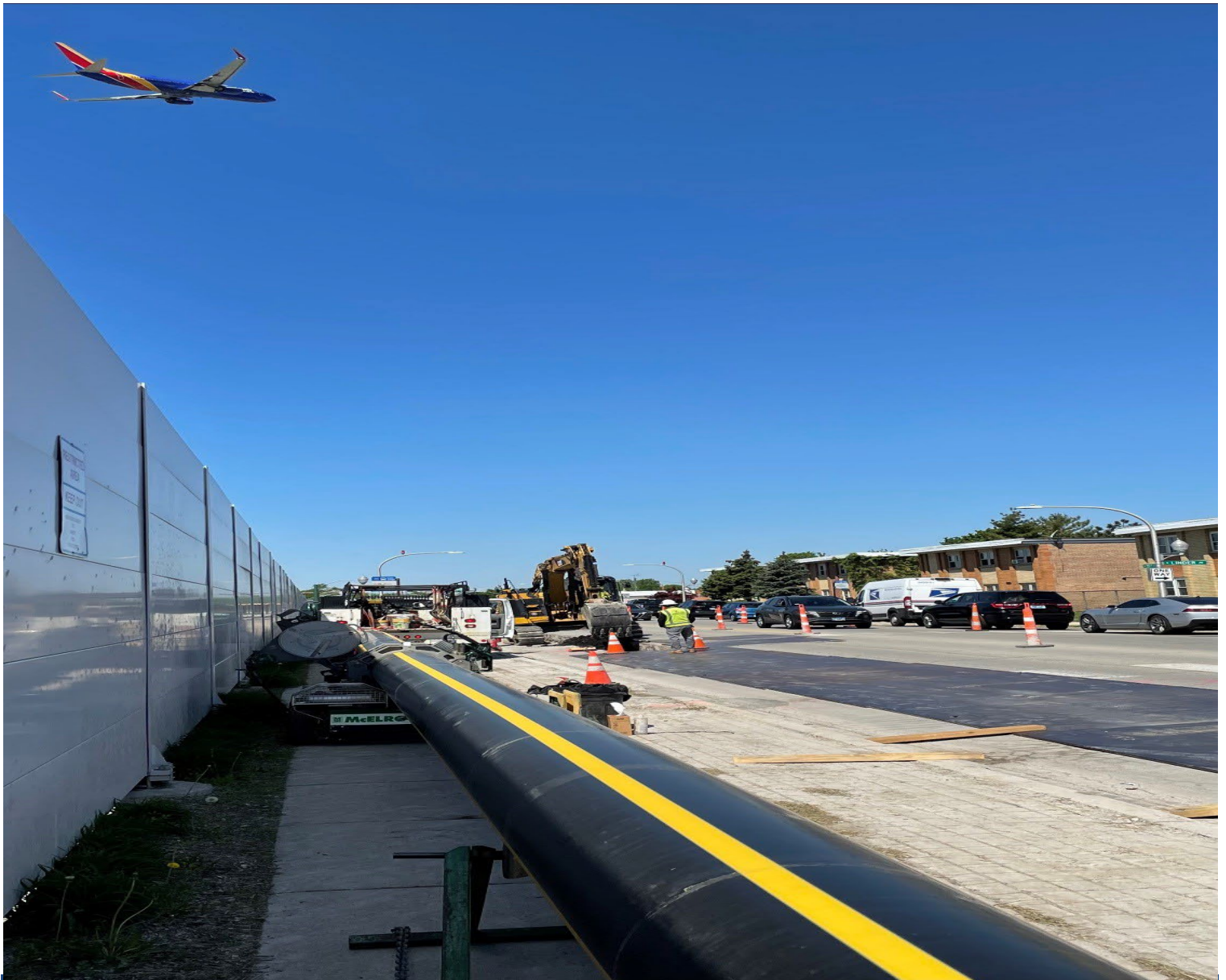
Garfield Ridge - 18" pipe being installed.
