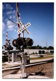
A frequent cause of highway-railroad grade crossing signal failures is vandalism. Police officers can assist by watching for trespassers or incidents of vandalism along the tracks, such as tampering with signal components (connecting wires, cables, lenses, switches, and cabinets). Crossing signals should also be observed for shattered lenses, burned out bulbs, and gate arm damage which could reduce warning effectiveness.
