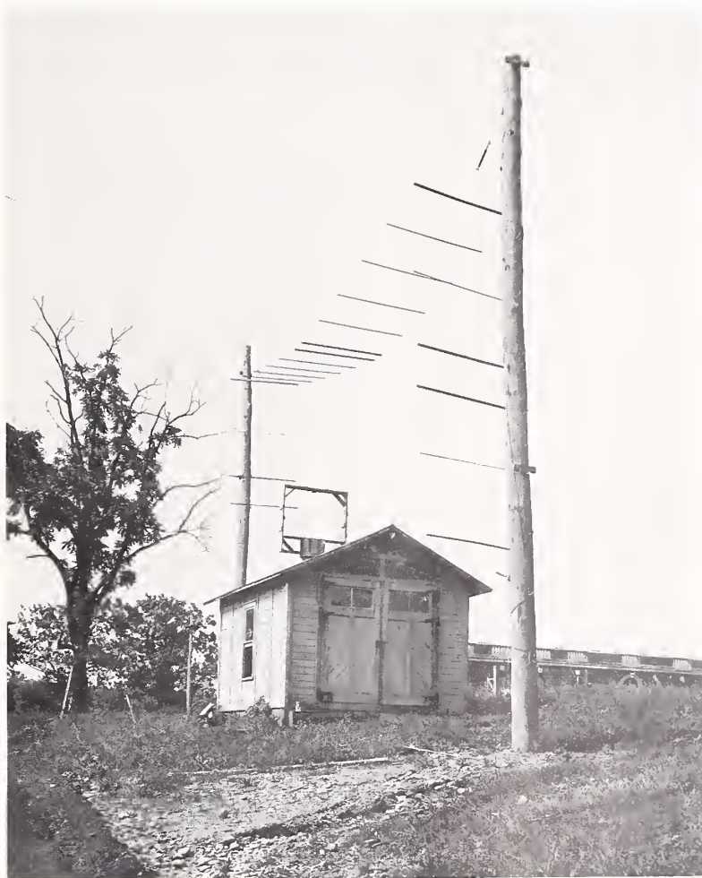
FIGURE 6—Special Type of Antenna for Transmission on 105 Meters, Consisting of 23 Turns in Parallel
