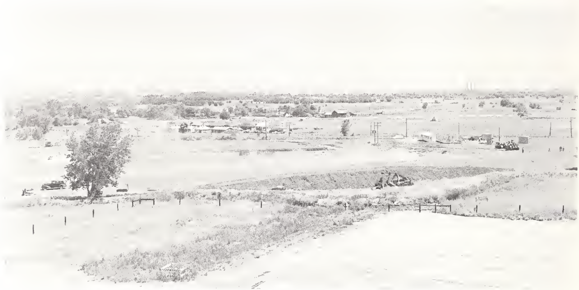
View of the area now occupied by the Radio Building, Boulder Laboratories, as it appeared on July 15, 1952, a few weeks after ground was broken for construction. The photo was taken in the vicinity of the present Plasma Physics Building (Building 24) and the view is in a northeasterly direction. The elevated grade of the Denver-Boulder Turnpike crosses the view nearly horizontally at mid distance. Early housing of Highland Park appears between the Turnpike and the nearer Marshall Road (now Broadway). Smokestacks of the Valmont Power Plant appear in the distance at right.
