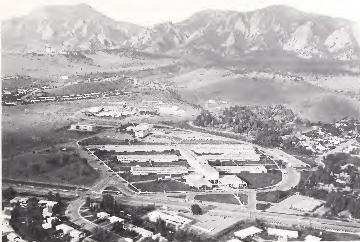
A 1973 view to southwest from helicopter over Highland Park subdivision east of Broadway (across lowest portion of photo). Spread across the middle portion of photo can be seen nearly the entire tract of the 217 acres of land on which have been constructed a number of buildings of the National Bureau of Standards at Boulder, Colo. In the foreground is the large Radio Building with six wings extending from the central spine.
