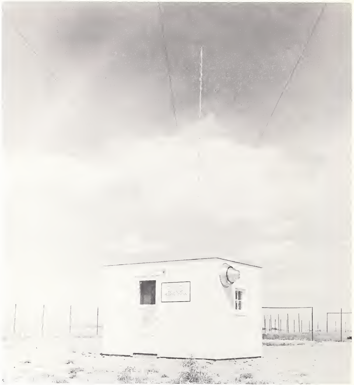
The NBS noise recording station located on Gunbarrel Hill northeast of Boulder, Colo. A whip antenna extends vertically above the center of an elevated ground plane consisting of wires radiating horizontally from the base of the antenna. Such a ground plane stabilizes the antenna impedance. This station was one of 16 scattered over the World for the IGY noise program of 1957-1958, 5 of the stations being operated by the NBS.
