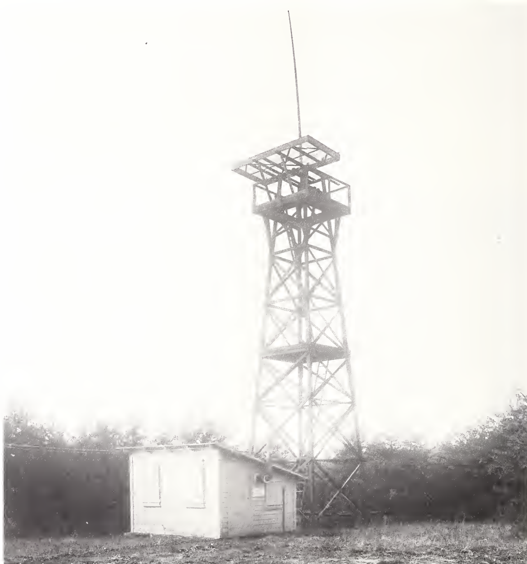
Building No. 2 and west antenna tower at Kensington, Md. field station. This building was used as a general laboratory and workshop area. Building No. 3 (not shown) housed the field-intensity recording equipment.
