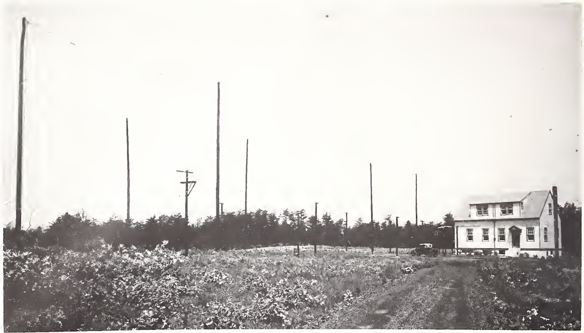
Transmitting building of station WWV used for the broadcasting of standard frequencies from December 1932 until destroyed by fire on November 6, 1940. This and other Radio Section buildings were located on the Experimental Farm of the Department of Agriculture, Beltsville, Md., northeast of Washington, D.C. Antennas and transmission-line feeders can be seen in the photograph.
