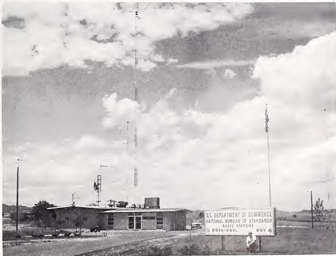
Administration wing and building that houses the 60-kHz transmitter and associated equipment of station WWVB, located near Ft. Collins, Colo. Antenna masts of the WWVL station (operated at 20 kHz) are in background.
