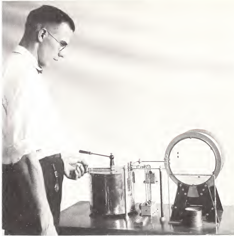
Richard T. Cox, who shared in improving the Bureau's standard wavemeter that became known as type R70B is shown making adjustments. Rods in fixed positions, used to connect the several components, minimized variation of calibrated values. This design, developed in 1920, served during the 1920's as the basic reference for other types of wavemeter standards. With four fixed mica capacitors and seven inductors, the wavelength range was 65 meters to 85,000 meters (4620 to 3.5 kHz).
