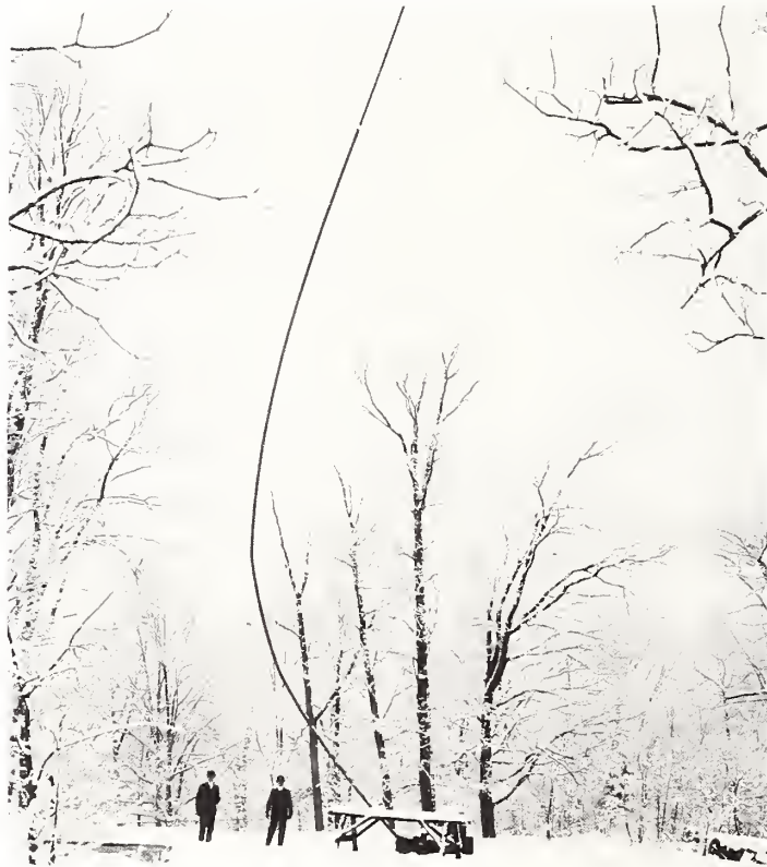
Antenna mast, buckled by a snowstorm of March 1914, was located to the east of the recently constructed East Building that housed the Bureau's radio laboratory. (Original print shows the arrays of guy wires "supporting" this mast.) It is the only known picture of a radio antenna associated with this laboratory.
