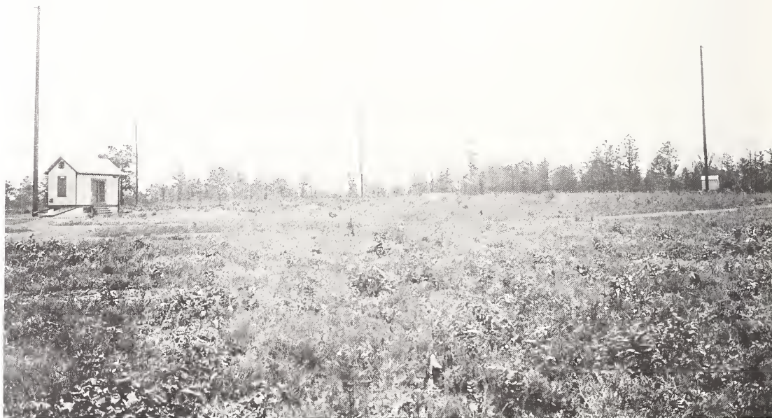
Beginning in 1932, this modest structure (Building No. 3) at the Beltsville, Md. field station provided the field laboratory for the Bureau's first automatic multifrequency ionosphere recorder that became the progenitor of all Bureau ionosondes that were to follow. The accompanying transmitter was also housed in this building. Later, the recorder was moved to the Meadows station.
