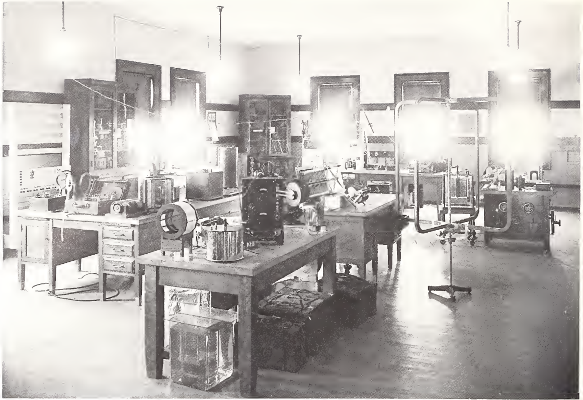
Wireless Laboratory, December 1915, located at north end of fourth floor, East Building. Many measurement instruments appear on the tables, including a standard capacitor and inductor, and Kolster receiver in center foreground. A two-coil direction finder is on the right.
