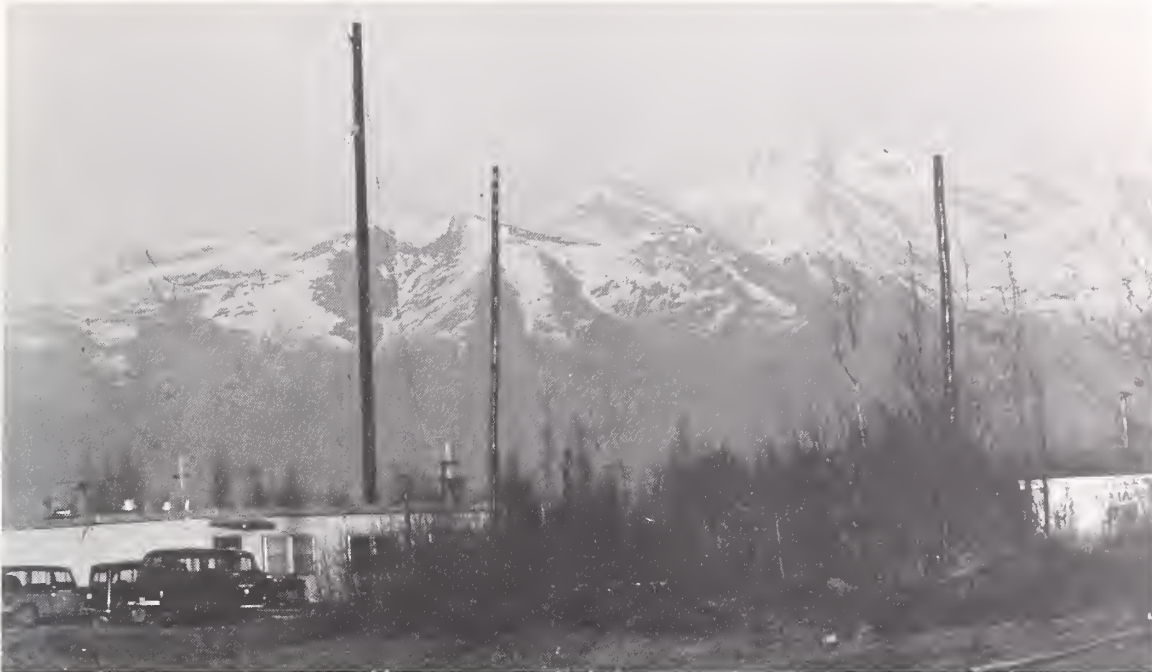
The Chugach Mountains form a backdrop to the North Pacific Radio Warning Station near Anchorage, Alaska, with operations beginning in 1951. The service covered radio communication paths extending from California through Alaska and across the Pacific to Japan. In 1964 the facility came and continues to be known as the High Latitude Space Environment Monitoring Station, now operated by NOAA (National Oceanic and Atmospheric Administration).
