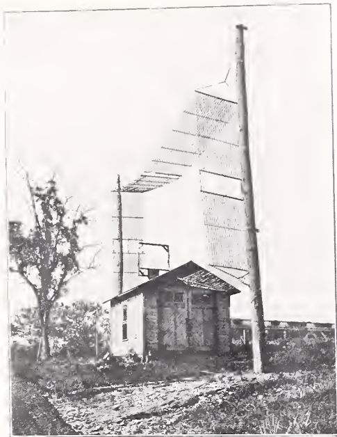
FIGURE 6—Special Type of Antenna for Transmission on 105 Meters, Consisting of 23 Turns in Parallel
