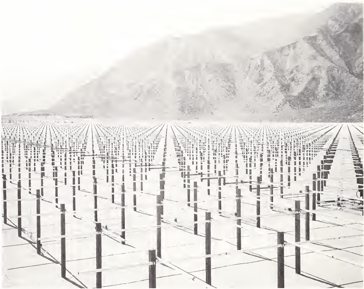
Dipoles by the thousands (9216 crossed pairs of half-wave dipoles)—covering an area of 21 acres—that serve as a huge antenna for a scatter radar installation. Construction of the facility, known as the Jicamarca Radar Observatory, began in January 1961 at Jicamarca, a site east of Lima, Peru, located near the geomagnetic equator. This venture into new realms of radio research of the ionosphere was a cooperative project of the Central Radio Propagation Laboratory and the Instituto Geofísico de Perú.
