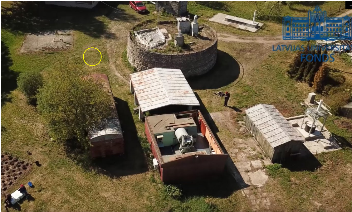
Figure 8-70. Riga station view: The SLR system, GNSS antenna, new local network markers (lower right, top right and near the GNSS antenna) and groundwater monitoring well (yellow circle). Between the SLR and the lower right marker is the old AFU-75 satellite photo camera shed.
