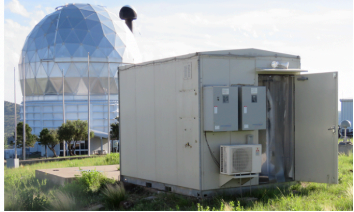
Figure 8-62. MGO gravimeter hut.
