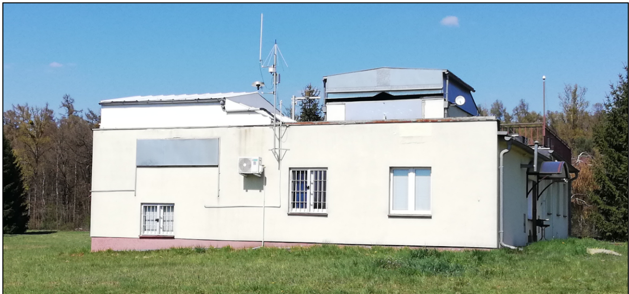
Figure 8-20. The Borowiec system building.
