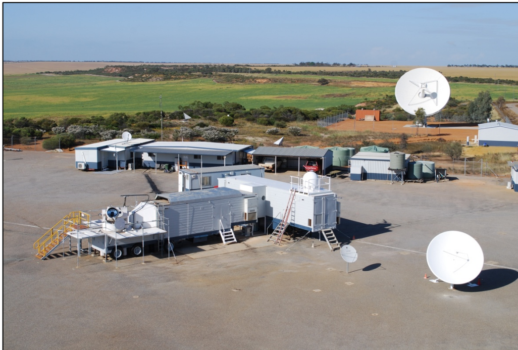
Figure 8-99. The Yarragadee Geodetic Observatory showing MOBLAS-5 vans with improved safety access, VLBI 12m antenna and two SAR calibration CRs.
